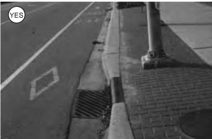
*Where space is tight but drainage requirements dictate an 18 in. (0.45 m) drain, a special 1 ft. (0.3 m) curbhead may be used with a 1 ft. (0.3 m) gutter pan (fig. 3-13).*
