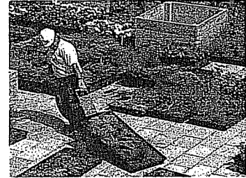
"greengrid" roof system installation
