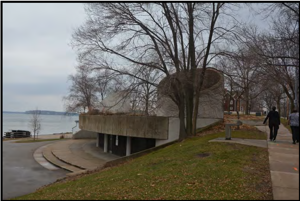
Figure Ten: Existing facilities showing graded areas in eastern Park area. View to east.
