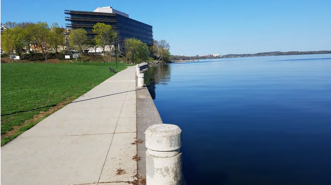
The majority of the shoreline is lined with a concrete wall.
