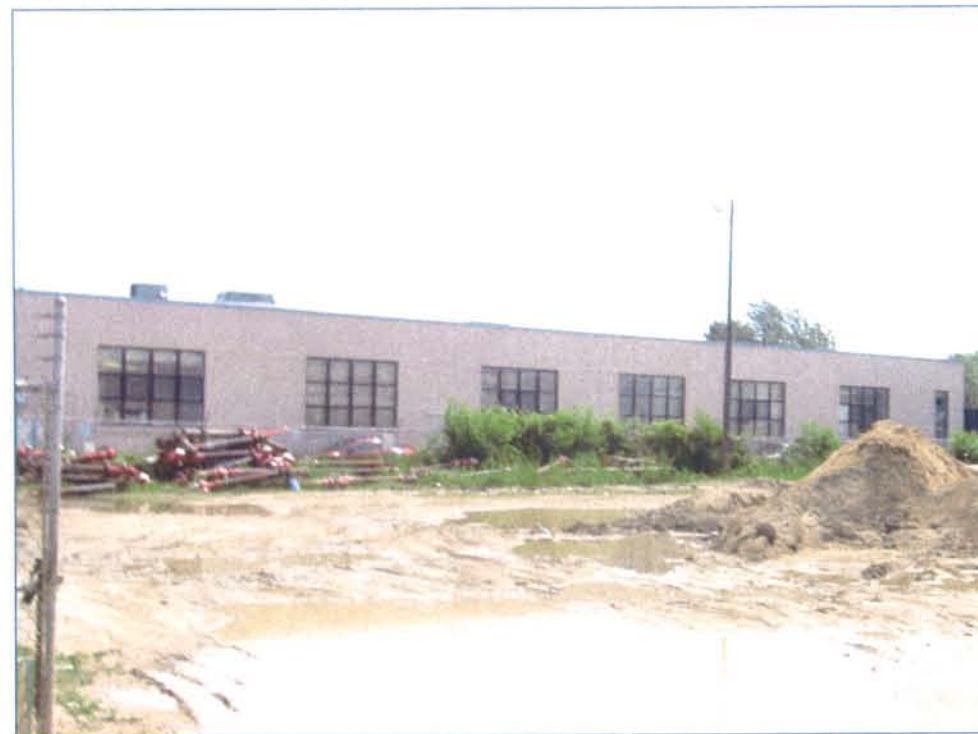
VIEW OF EAST SIDE OF LOT
