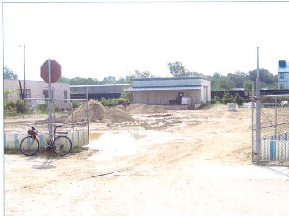
VIEW OF ENTRY FACING SOUTH
