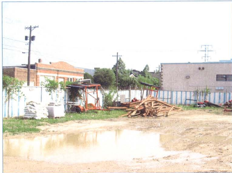
VIEW OF NORTHEAST PORTION OF LOT
