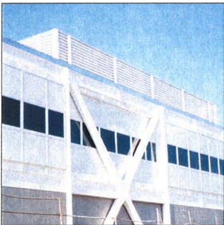
ID 4282 – Puente Learning Center, Los Angeles, CA Contractor: Swinerton & Walberg, Los Angeles CA Custom sound reduction LiteWall providing high acoustical properties of nominal 40 STC for site near LAX airport.
