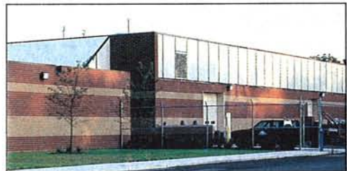
ID 3783 – Springfield City Service Complex, Springfield, OH Architect: Kevin Porter Assoc., Dayton, OH Contractor: Monarch Construction Co., Cincinnati, OH One 10' x 890' Wall Light and two 7' x 118' Wall Lights, both glazed in self supporting 3" Quadwall®. Glazing Colors: 8mm White 60 over 8mm White 60.
