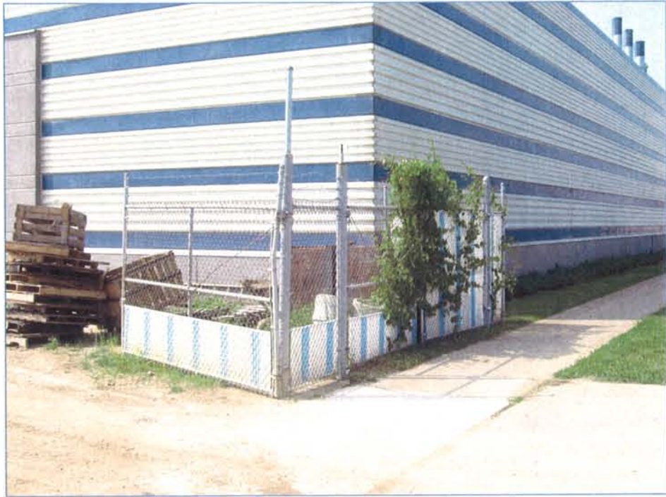
VIEW OF ENTRY FACING WEST
