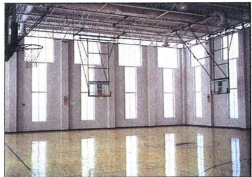
ID 4368 – Green YMCA, Greensburg, OH Architect: GPD Associates, Akron, OH Contractor: Wely Building Corporation, Akron, OH 26 Self Supporting Wall Light units, 250 linear feet by up to 25' high, glazed in 3" Quadwall®. Glazing Colors: 8mm White 60 over 8mm White 60.
