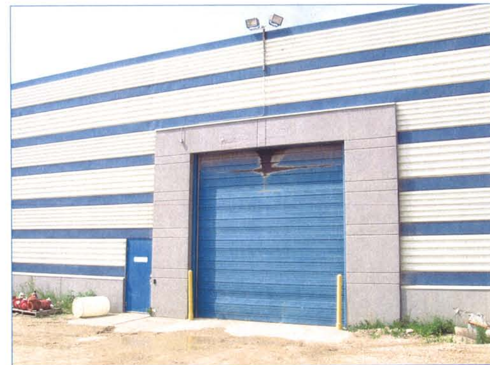
VIEW OF ENTRY DOOR FOR VEHICLE STORAGE
