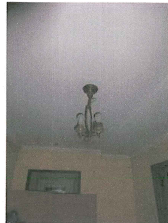
Image 10 Original light fixture, main entry, first floor
