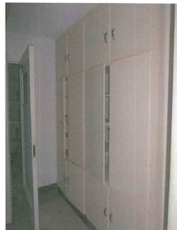
Image 8 Built in cabinets, first floor
