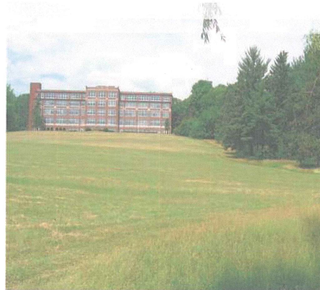
View to the Main Sanatorium from Northport. Dormitory for Help is shielded from view by trees and shrubs
