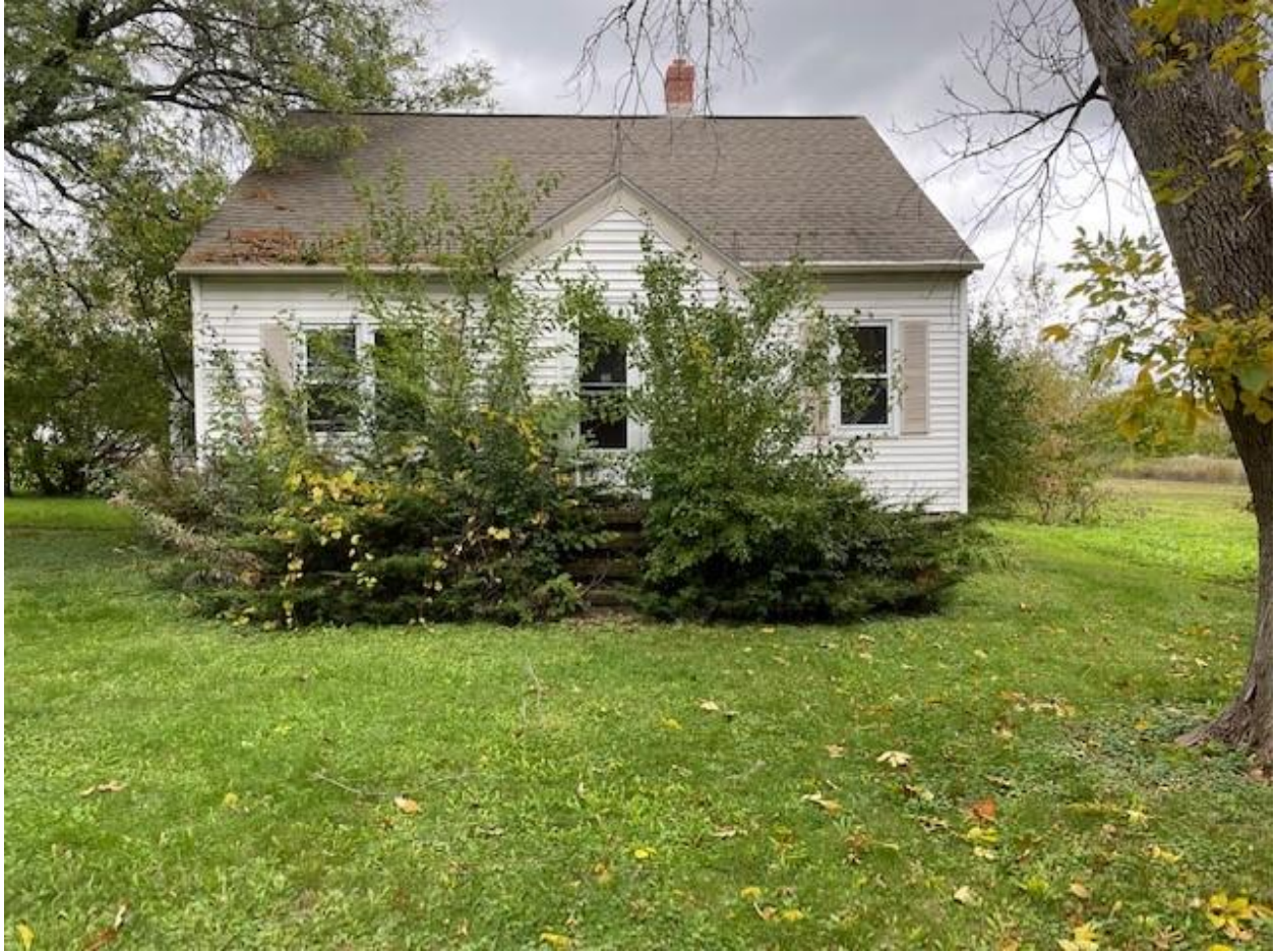
Figure 3: House exterior (facing North).
