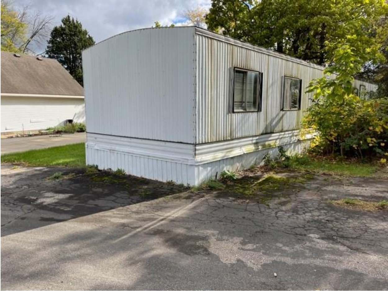
Figure 19: Mobile home exterior (facing South/East).
