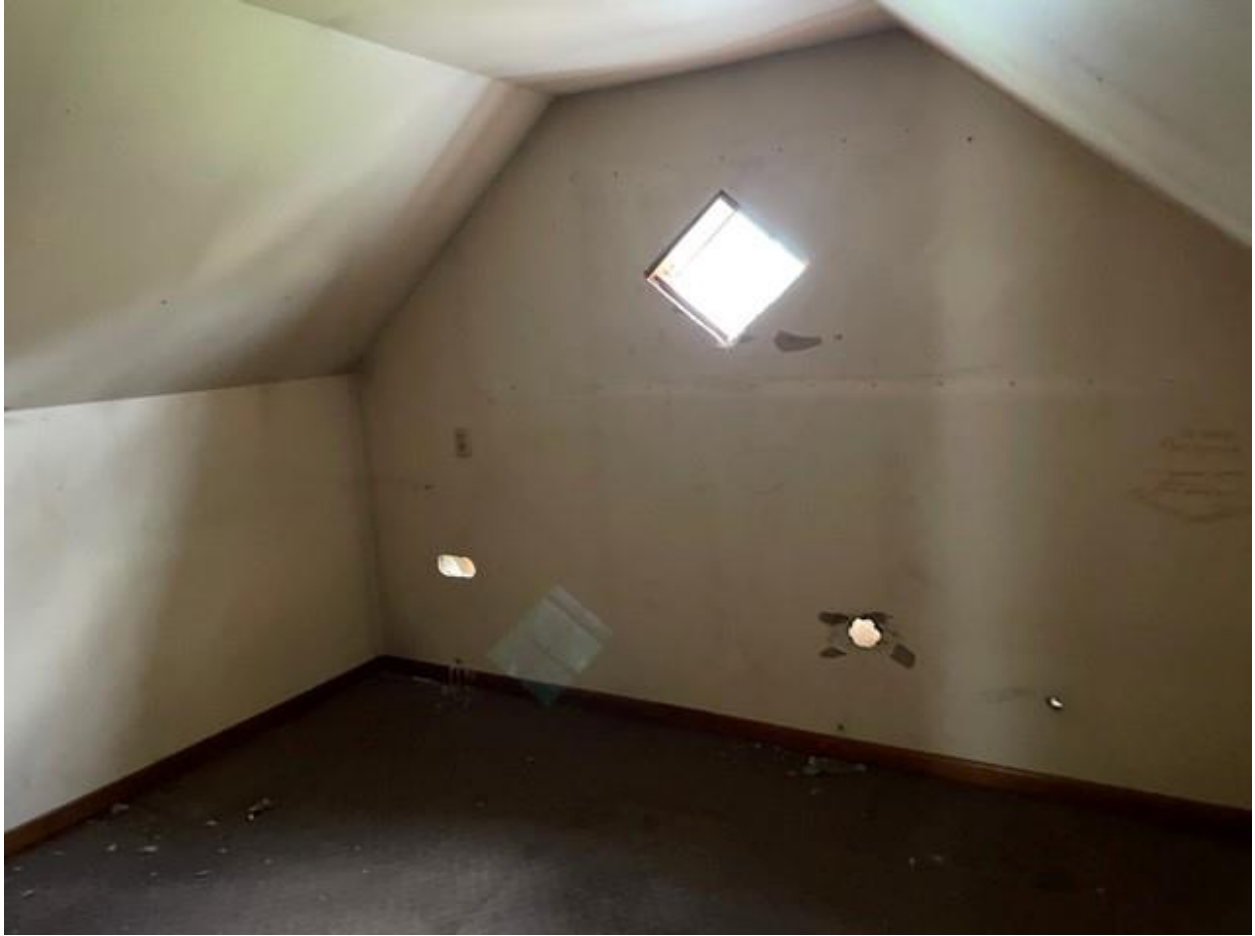
Figure 16: Garage interior (upper level).
