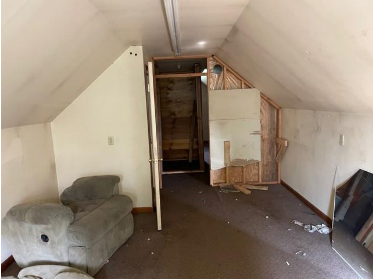
Figure 18: Garage interior (upper level).
