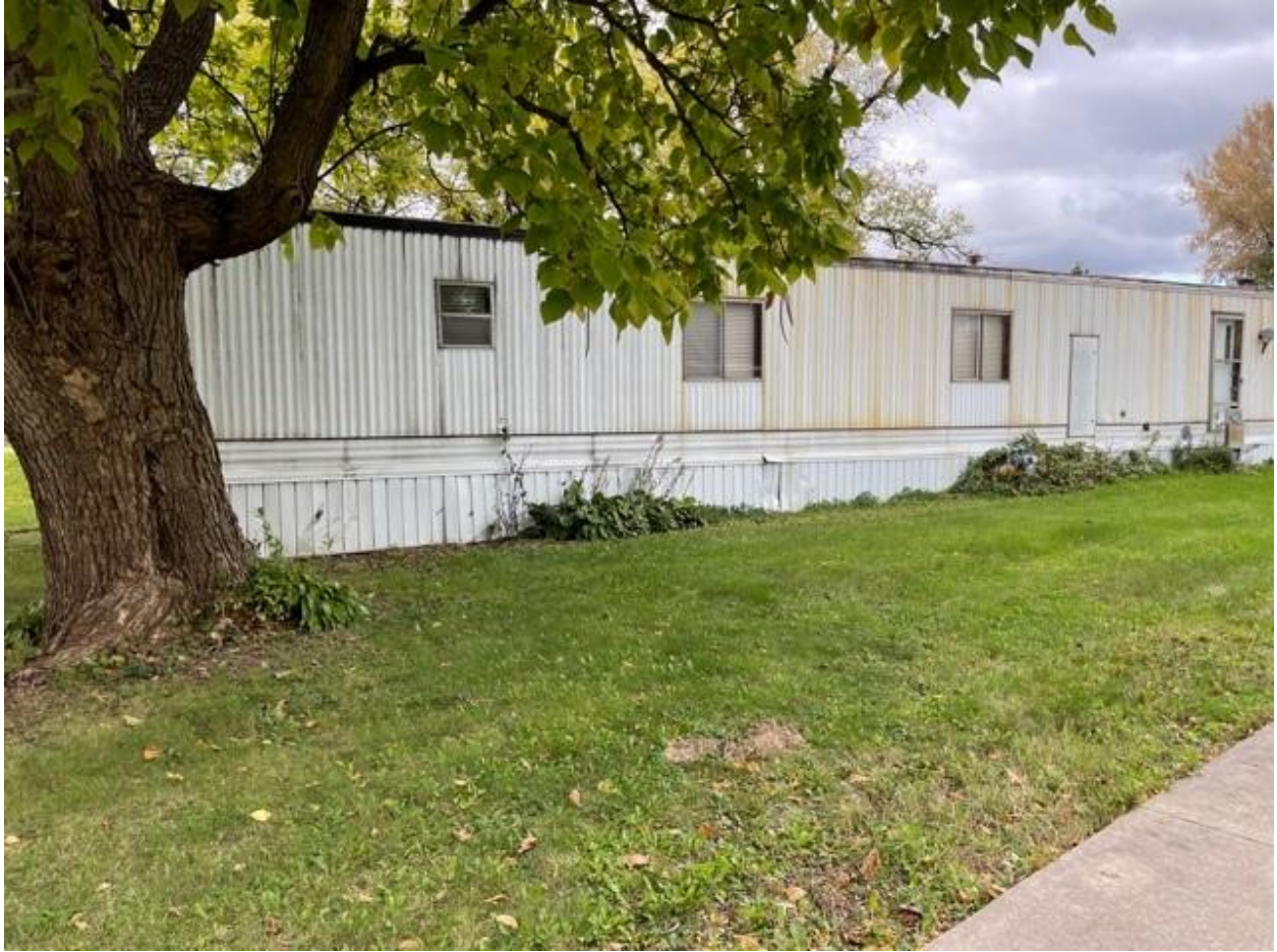
Figure 23: Mobile home exterior (facing West).
