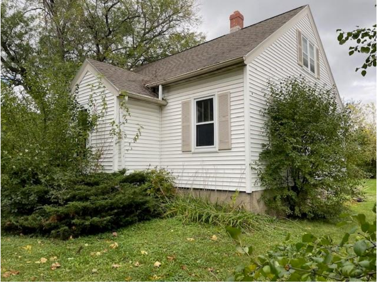
Figure 4: House exterior (facing North/West).
