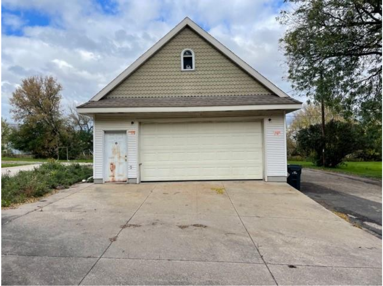
Figure 13: Garage exterior (facing North).
