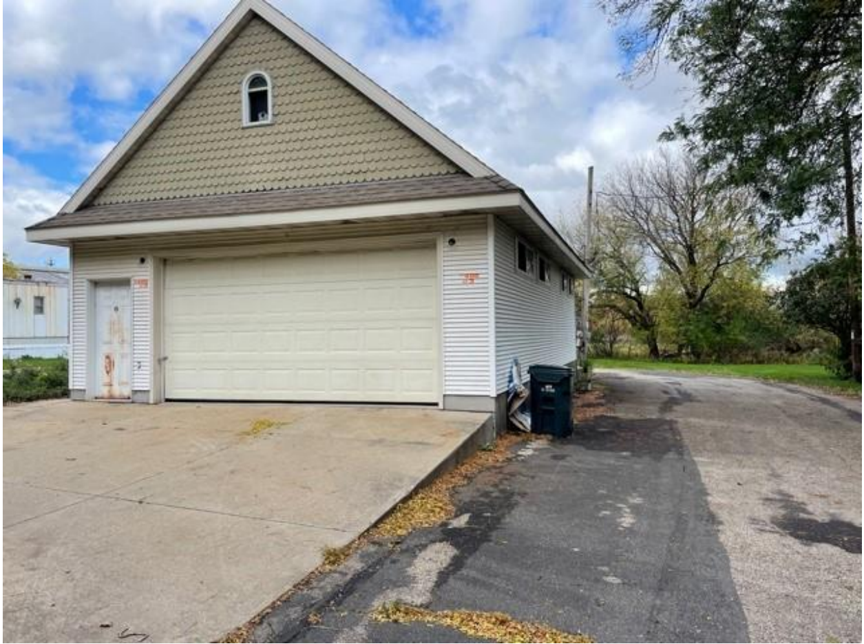
Figure 14: Garage exterior (facing North/West).
