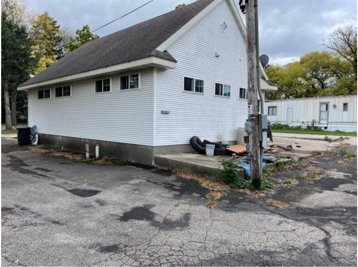
Figure 10: Garage exterior (facing South/West).
