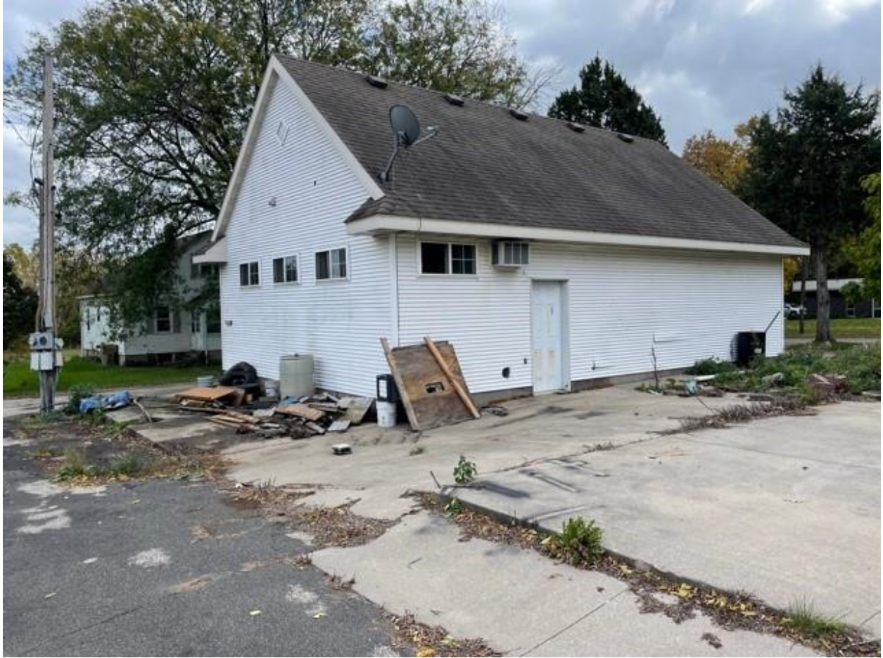
Figure 11: Garage exterior (facing South/East).
