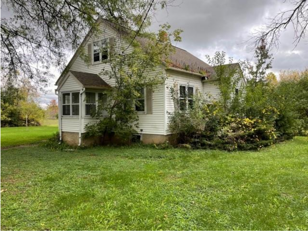
Figure 2: House exterior (facing North/West).
