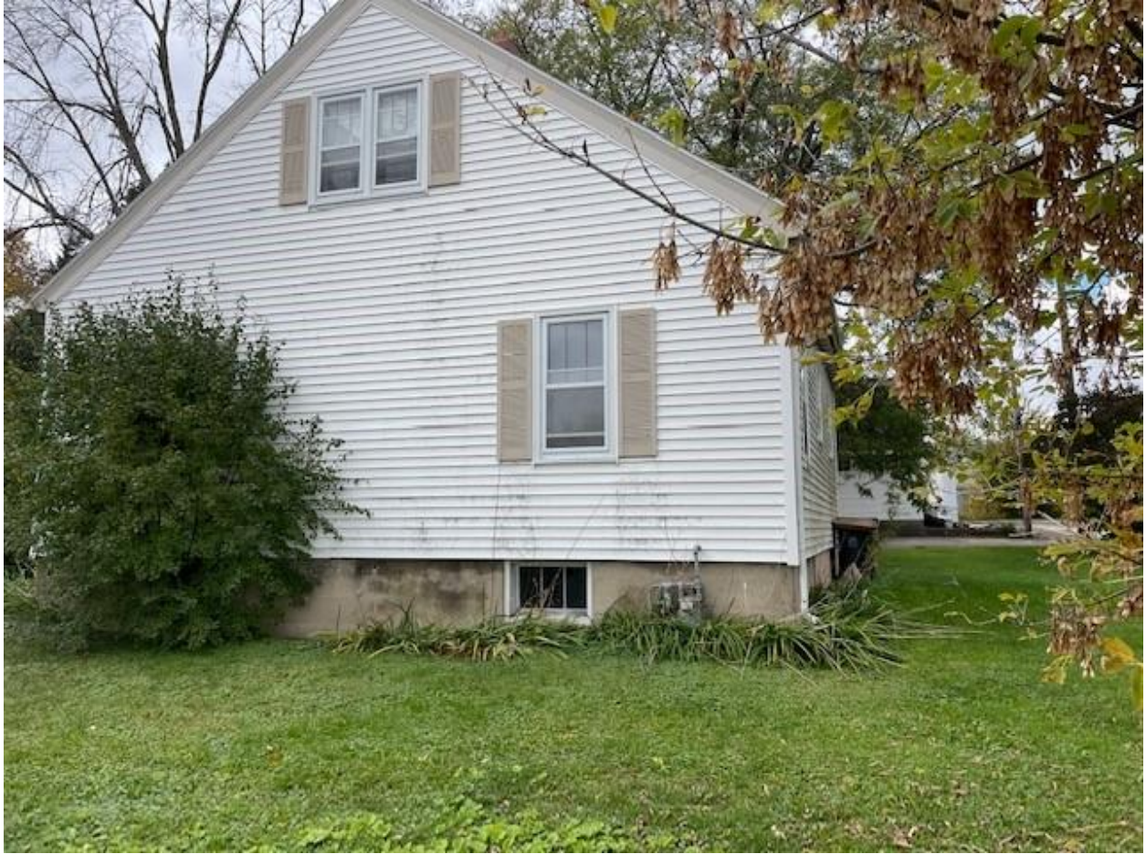
Figure 5: House exterior (facing South).
