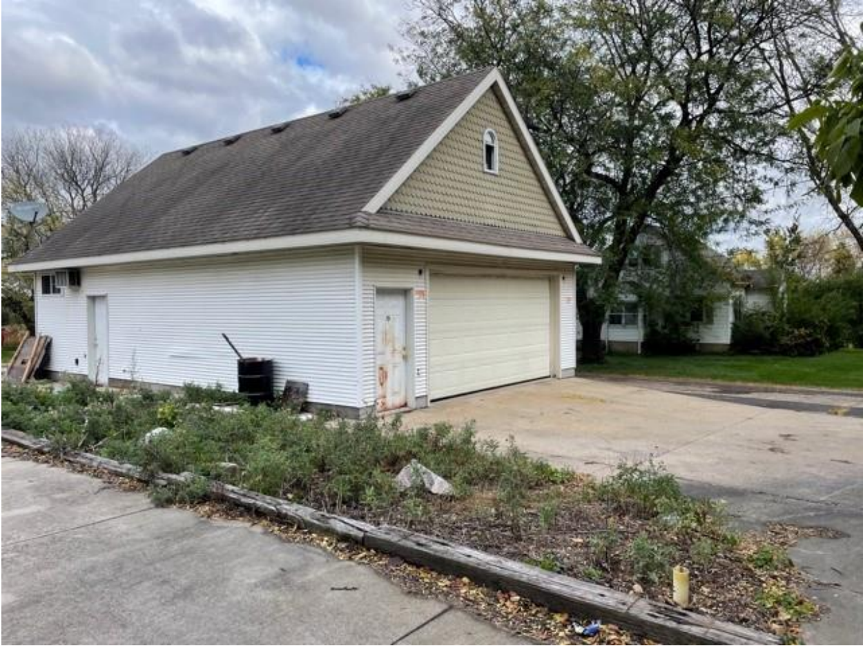
Figure 12: Garage exterior (facing North/East).
