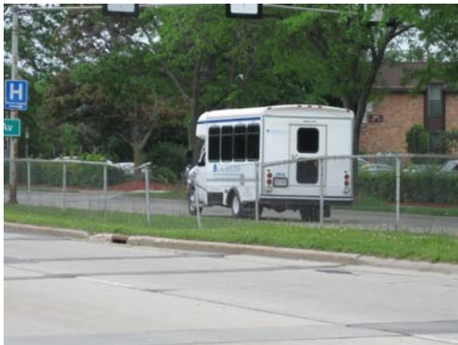
Broken fence in median, Northport Drive near Dryden Drive
