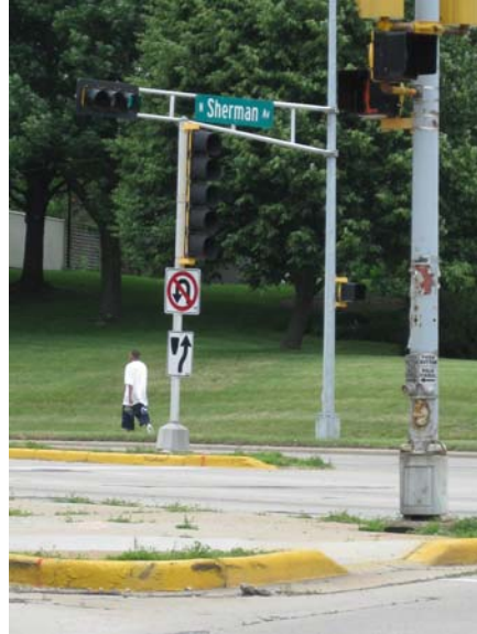
Weedy medians, rusty poles, Northport Drive at Sherman Ave.
