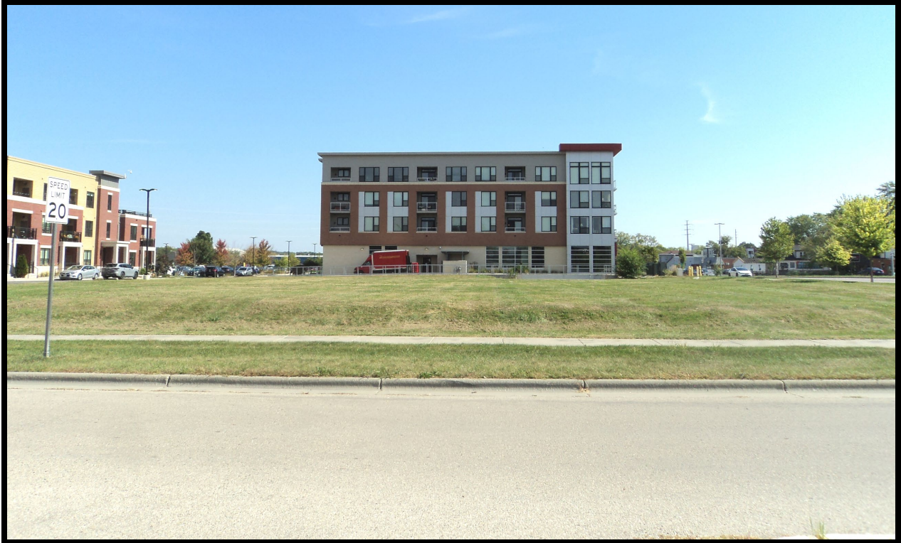
View of the Parcel at 501 Grand Oak Trail Looking East from Royster Oaks Drive
