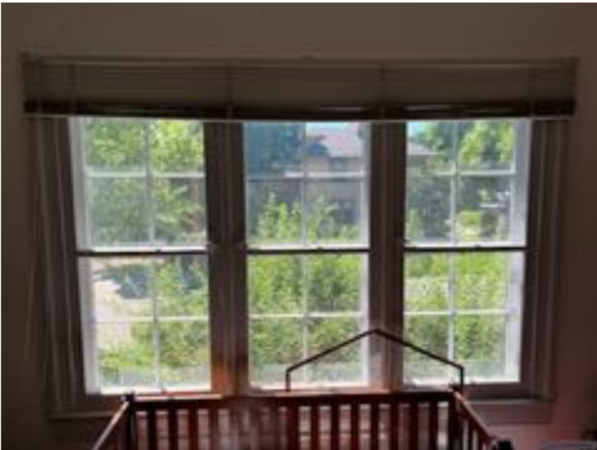
Window #2 – Interior view of 3-wide casement.
