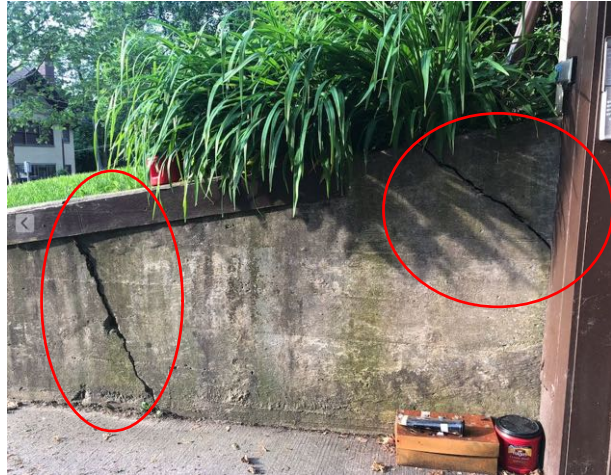
STRUCTURAL FAILURE OF THIS WALL
