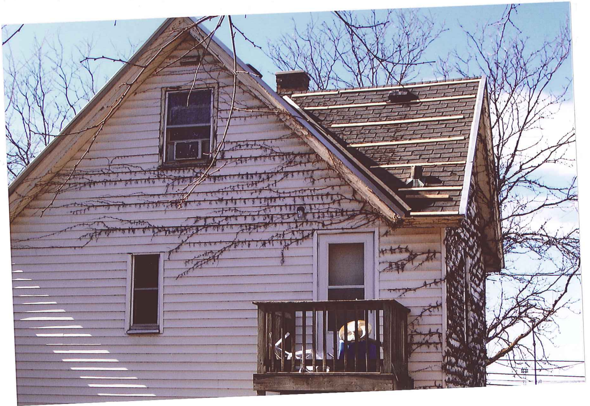
At the moment (as a result of our inability to raise the cash to remove the metal roof (that is 80% complete and paid for) and
