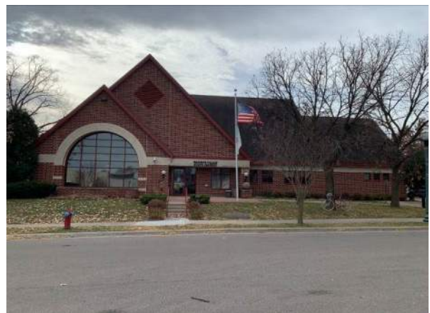
Photo 6: East-adjacent Madison Police Department – South Station at 825 Hughes Place. Photo facing south.
