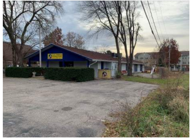
Photo 2: Overview of Site facing southeast from Hughes Place.
