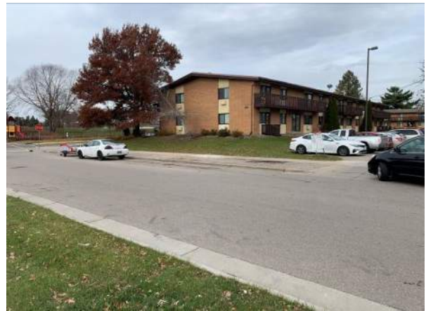
Photo 4: Overview of northwest-adjacent property, Oakridge Apartments, at 2317 Cypress Way. Photo facing northwest.
