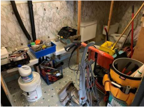
Photo 13: Maintenance and cleaning room in the center of the building.
