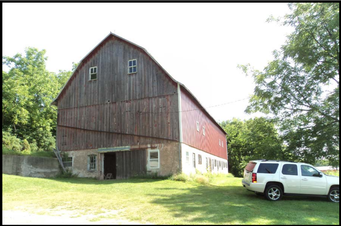
Main Barn – Exterior View
