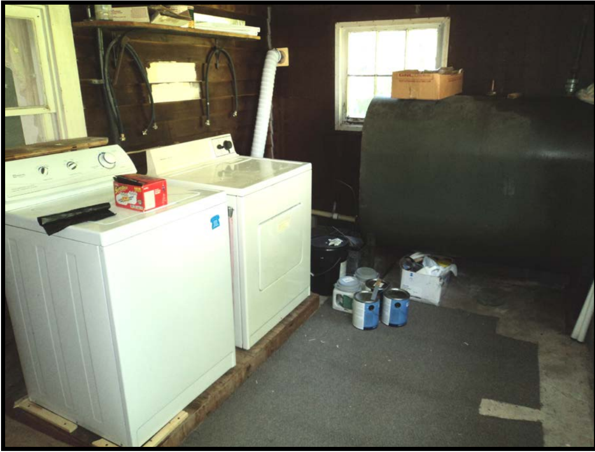
Single Family Residence – Laundry/Utility Room
