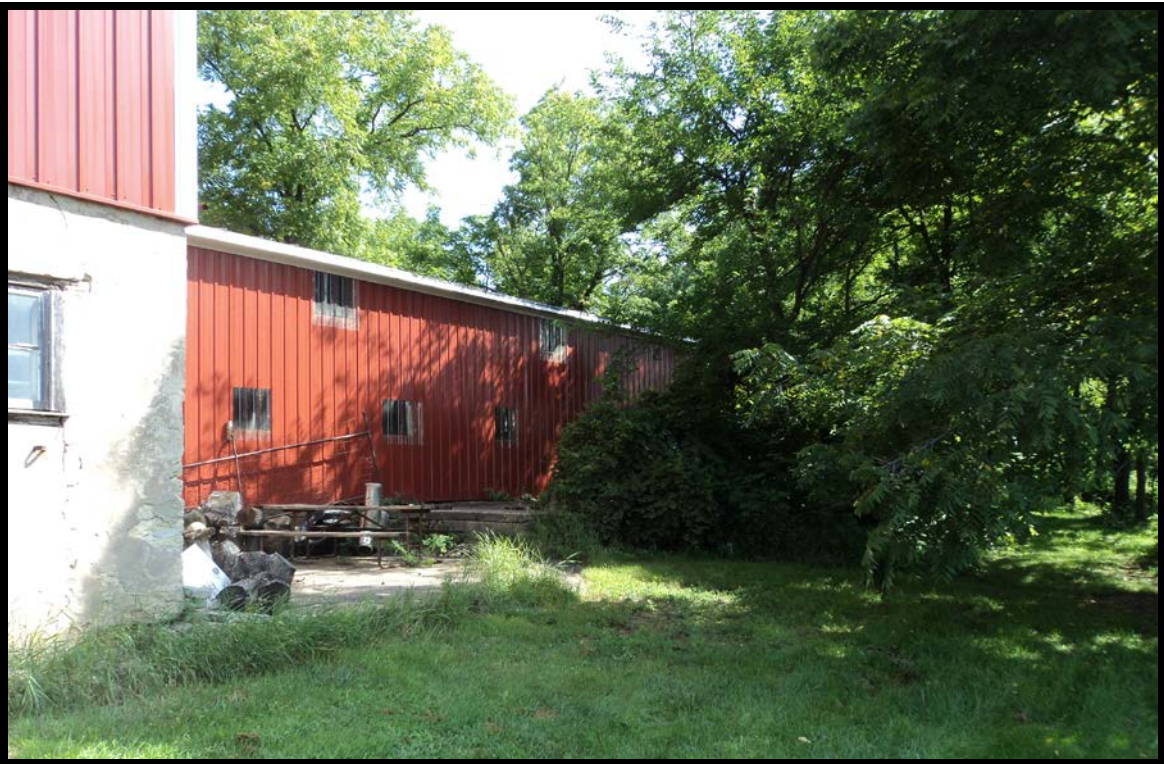
Attached Feeder Barn – Exterior View
