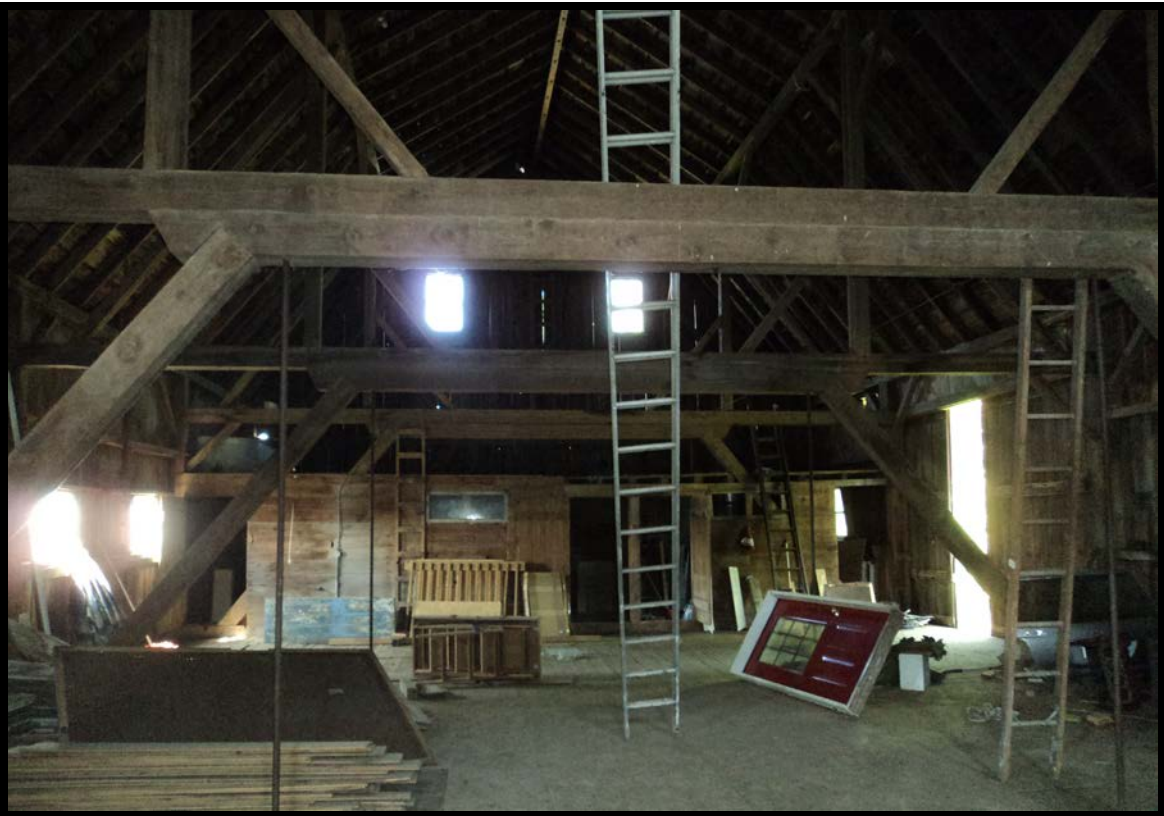
Main Barn – Second Story Interior View
