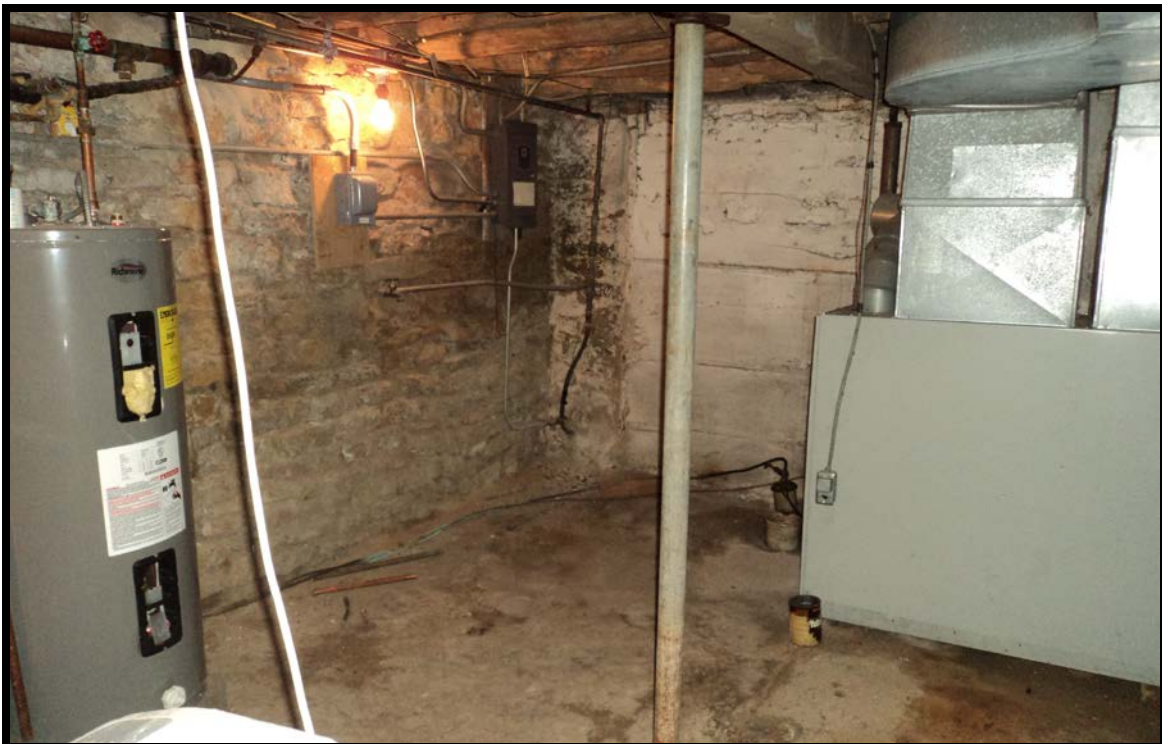
Single Family Residence – Unfinished Basement
