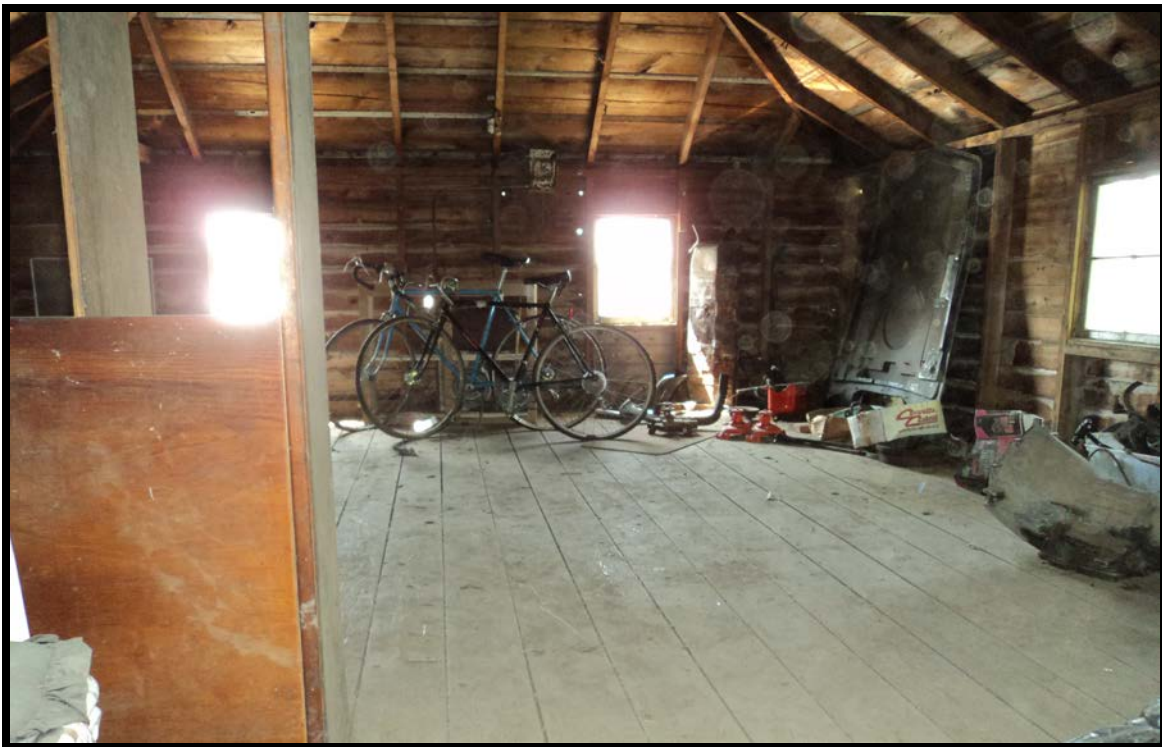
Detached Garage – Interior View of the Upper Level
