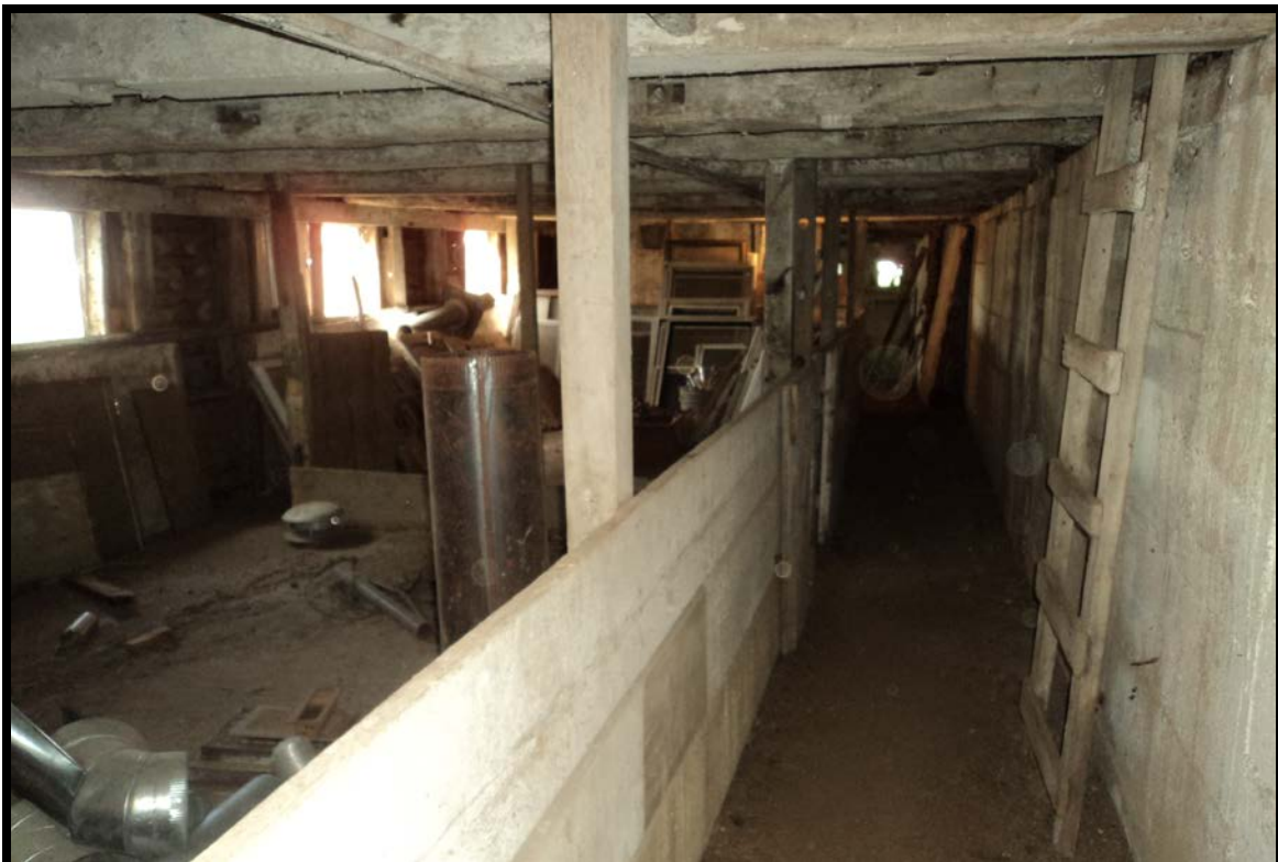
Feeder Barn – Interior View
