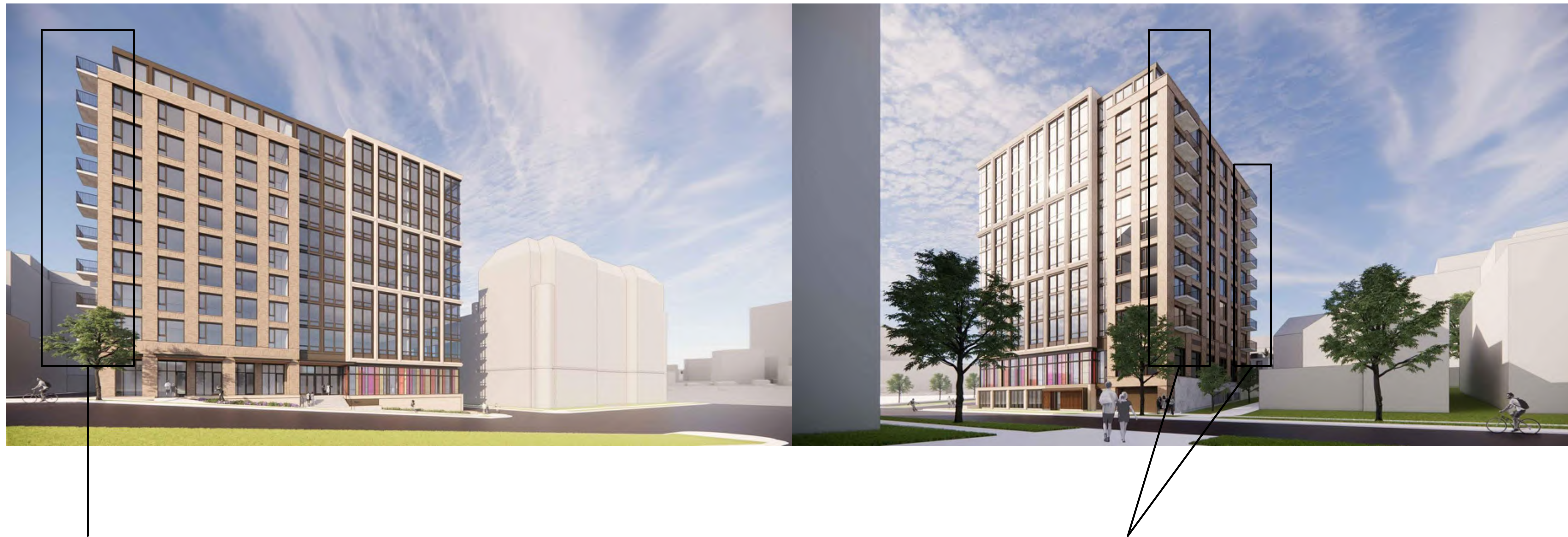
Fixture type EL13 installed recessed in the wall under the concrete structure of each of the private terraces. Light distribution will be indirect with complete concealment of light source by the extent of the terrace.
