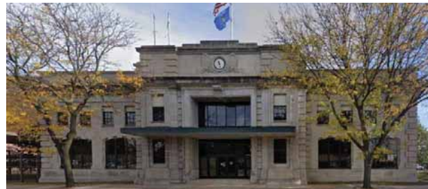
631 RAILROAD ST. FLAT ROOF, MASONRY, DOUBLE-HEIGHT ENTRY EXPRESSION, BASE WAINSCOT, CORNICE EXPRESSION, WINDOW GROUPINGS, RELATIVE SCALE, BEAUX ARTS STYLE, ARCHED WINDOWS
