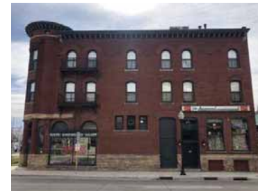
524 E. WILSON ST. FLAT ROOF, MASONRY, BASE WAINSCOT, WINDOW PROPORTIONS, RELATIVE SCALE, ARCHED WINDOWS
