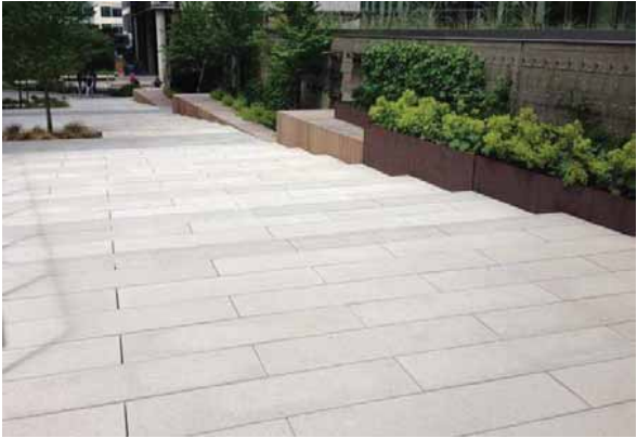
DRIVE ISLE LARGE SCALE RUNNING BOND PATTERN
