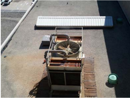
Figure 31 – Cooling Tower Condition
