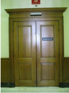
Figure 28 – Quarter Sawn White Oak Doors and Frames leading into Room 260
