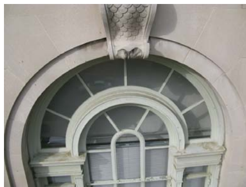
Figure 13 – Windows are Framed with Decorative Cast Iron, Sashes are Steel.
