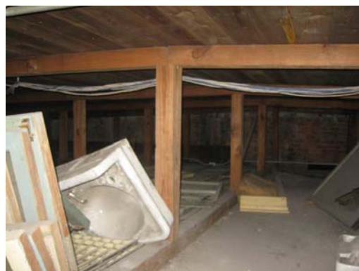
Figure 55 – Underside of Pitched Wood Roof Framing
