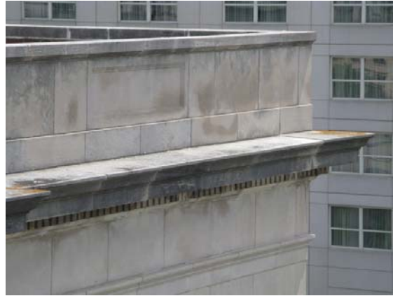
Figure 9 – Stone Cornice and Parapet
