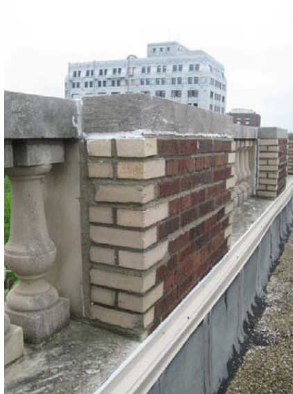
Figure 62 – Brick and Stone Parapet
