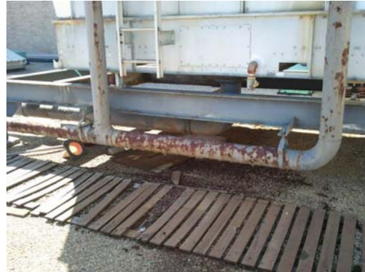
Figure 32 – Cooling Tower Condition
