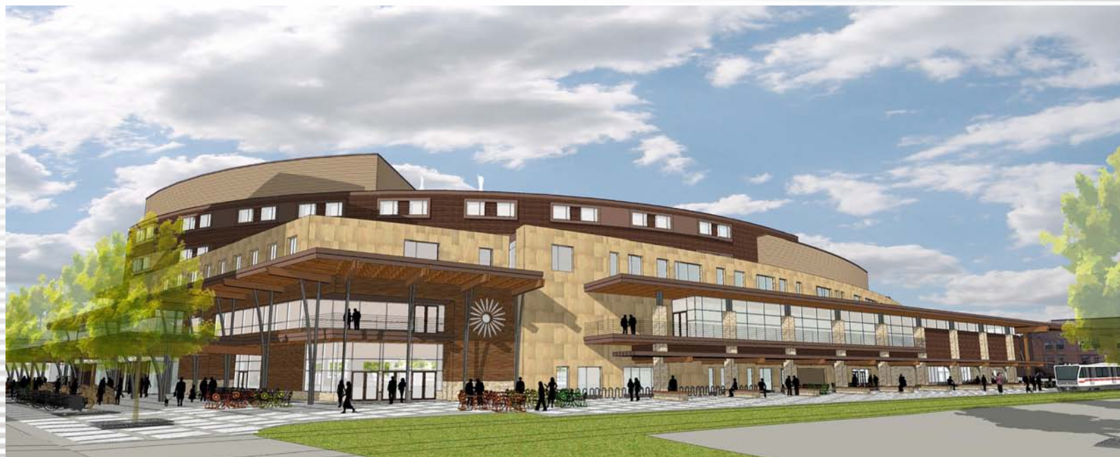
1. NORTH ELEVATION VIEW
