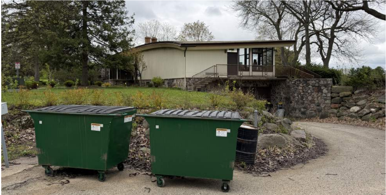
North elevation of Clubhouse. Garage door access at basement level.
