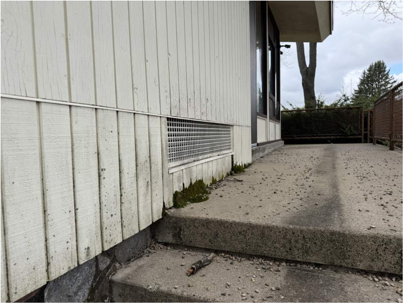
Detail of wall condition at North elevation.
