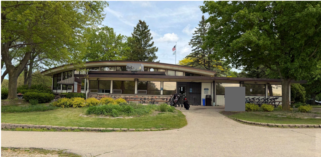
West elevation of the Clubhouse showing the windows and patio that overlook the golf course.
