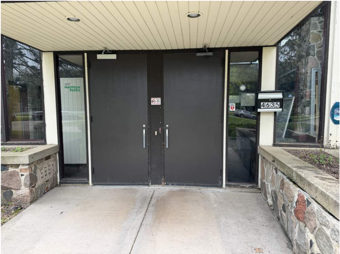
Detail of entrance on East elevation.
