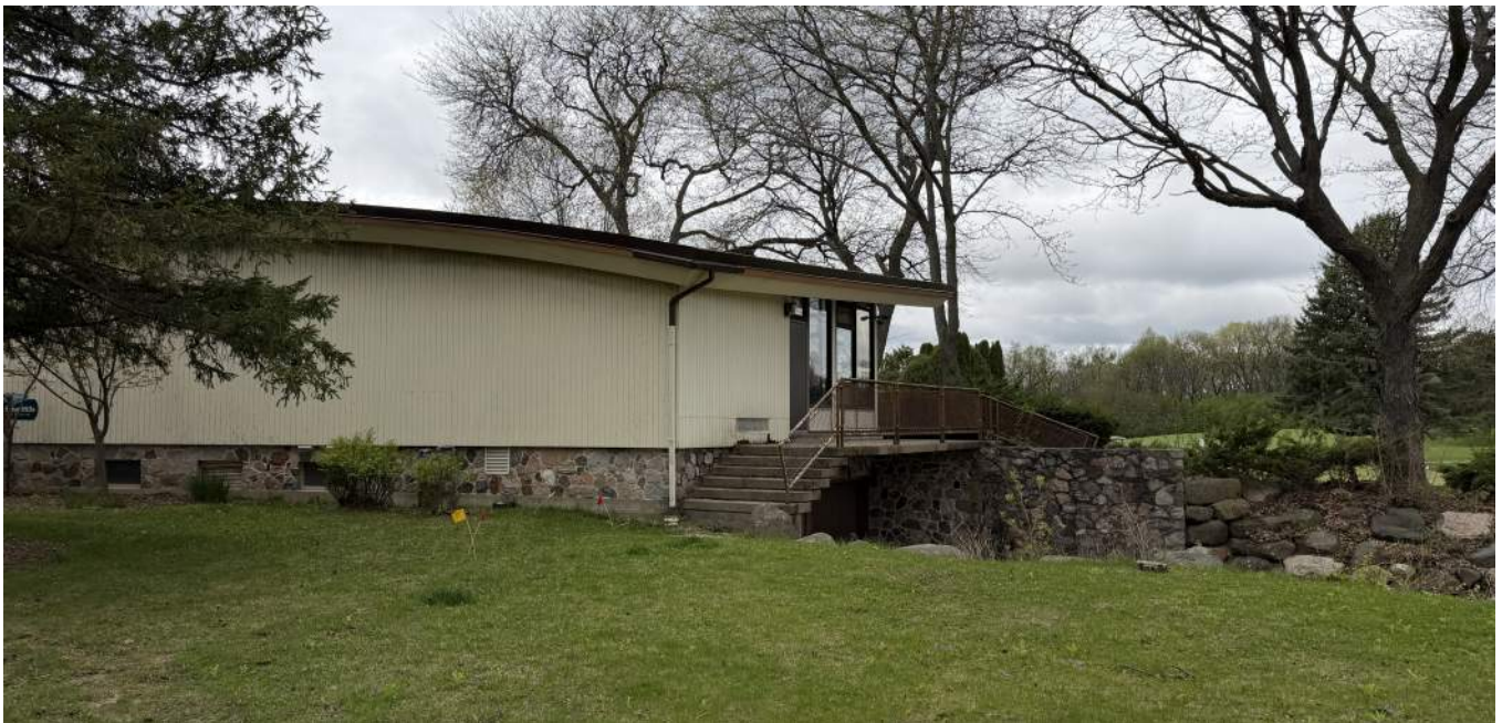
View showing the North end of the front and North elevation of Clubhouse.
