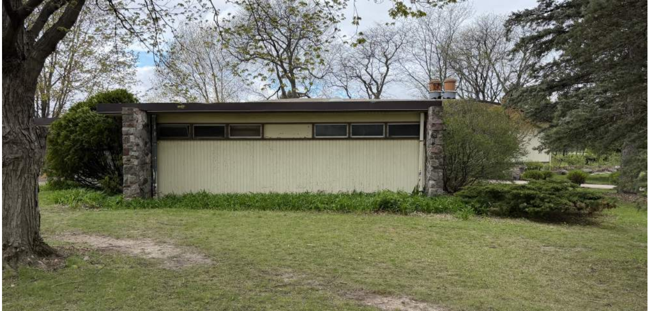
South elevation of Clubhouse.
