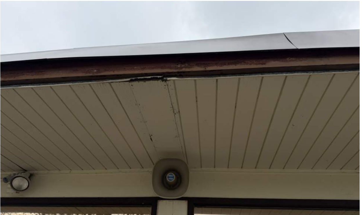
Detail of soffit and fascia condition.
