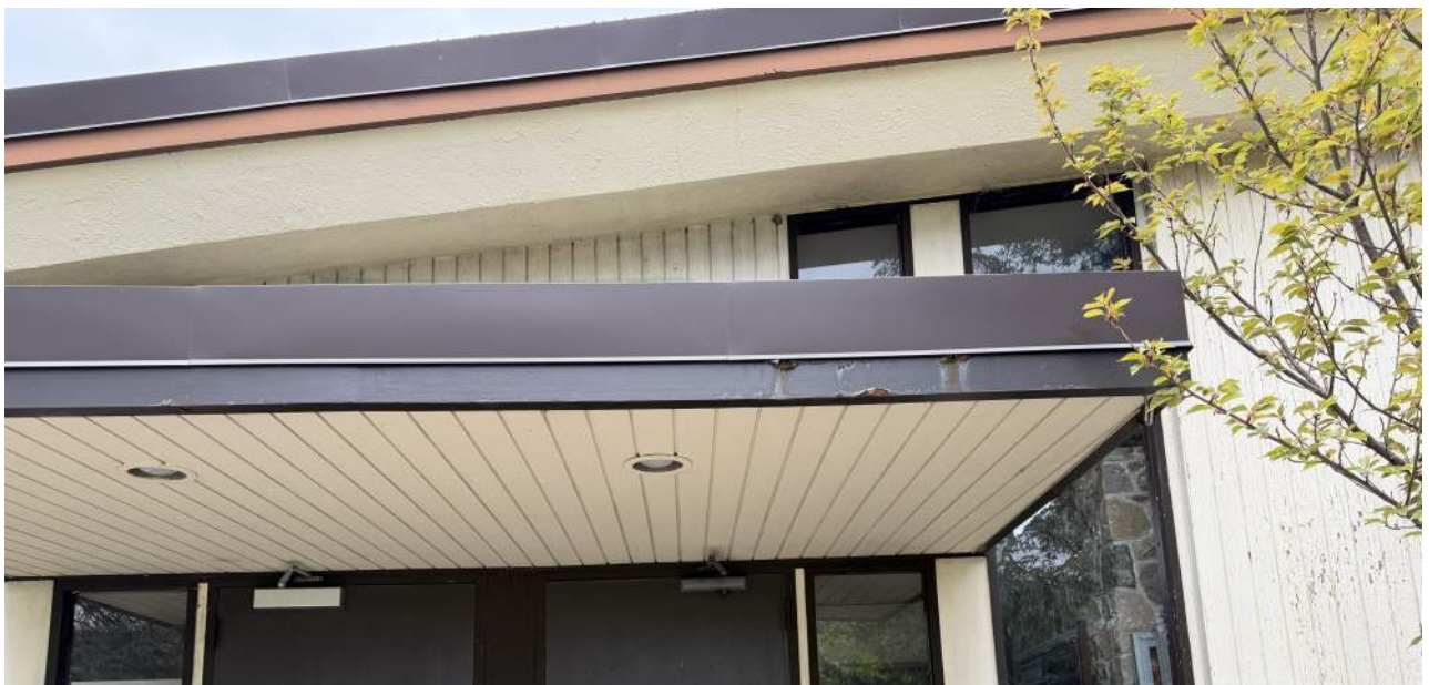
Detail of entrance overhang condition.
