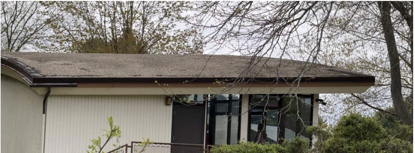
Detail of roof condition.
