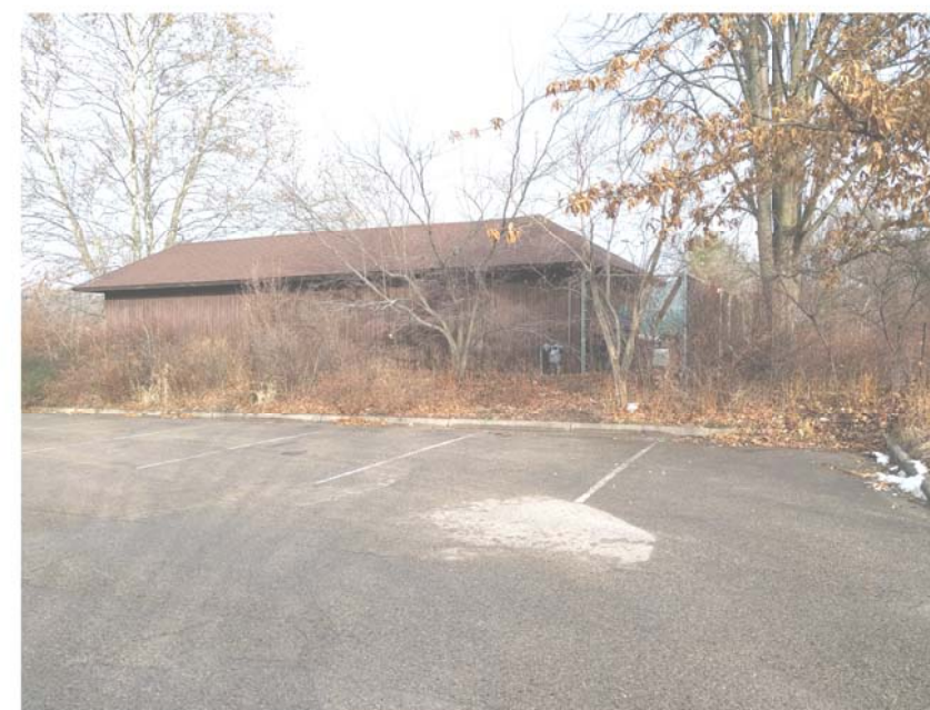
Existing Maintenance Shed
