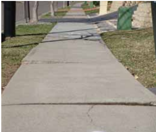
Fig 2.1.4 - Pavement damage caused by shallow rooting.
