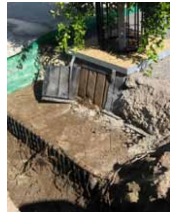
Trees with aggressive root systems have been planted in GreenBlue root management and soil cell systems, and excavated for research.
