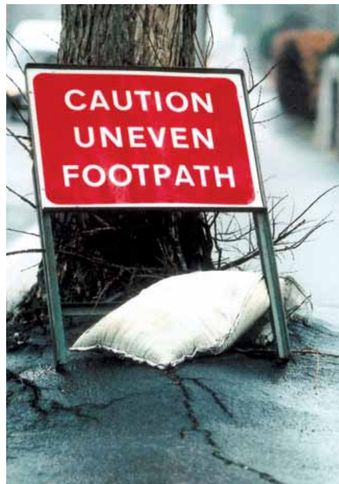
Fig 2.1.1 & 2.1.2 - Trees are frequently observed in cities either failing in the face of hostile growing conditions, or surviving and causing damage to pavements.
