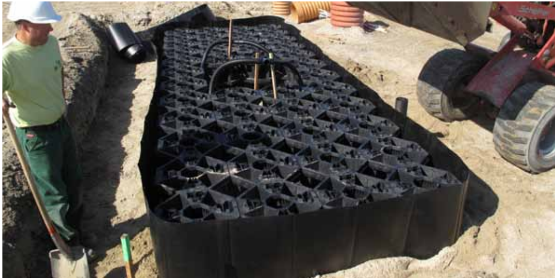
Strata Cell® modular system is fast to install, and ideal for provision of large soil volumes (94% of total pit volume) beneath paved surfaces.
