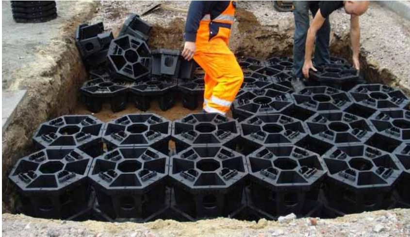
Fig 2.3.16 - Assembling High Strength Structural Soil Cells in Scandinavia
