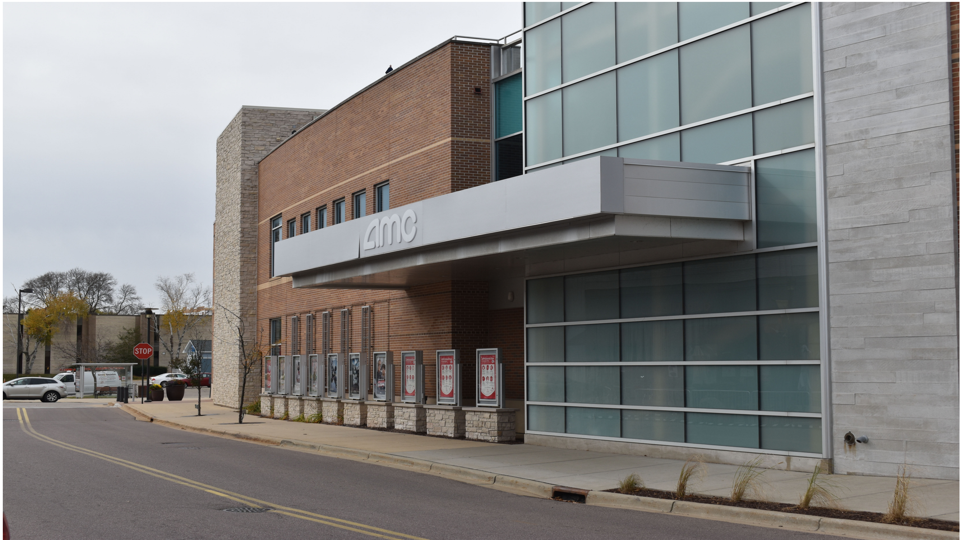
BUILDING 100 - SOUTHEAST PHOTO OF EXISTING
