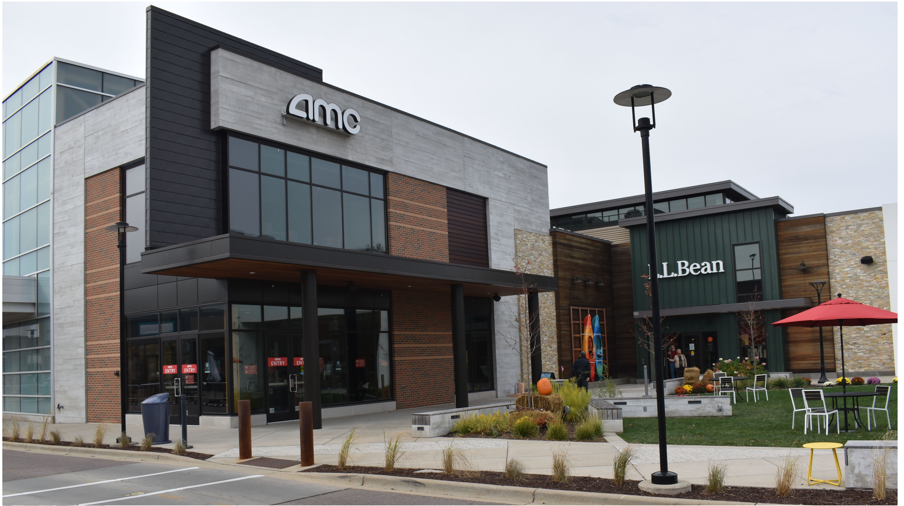
BUILDING 100 - SOUTHEAST PHOTO OF EXISTING
