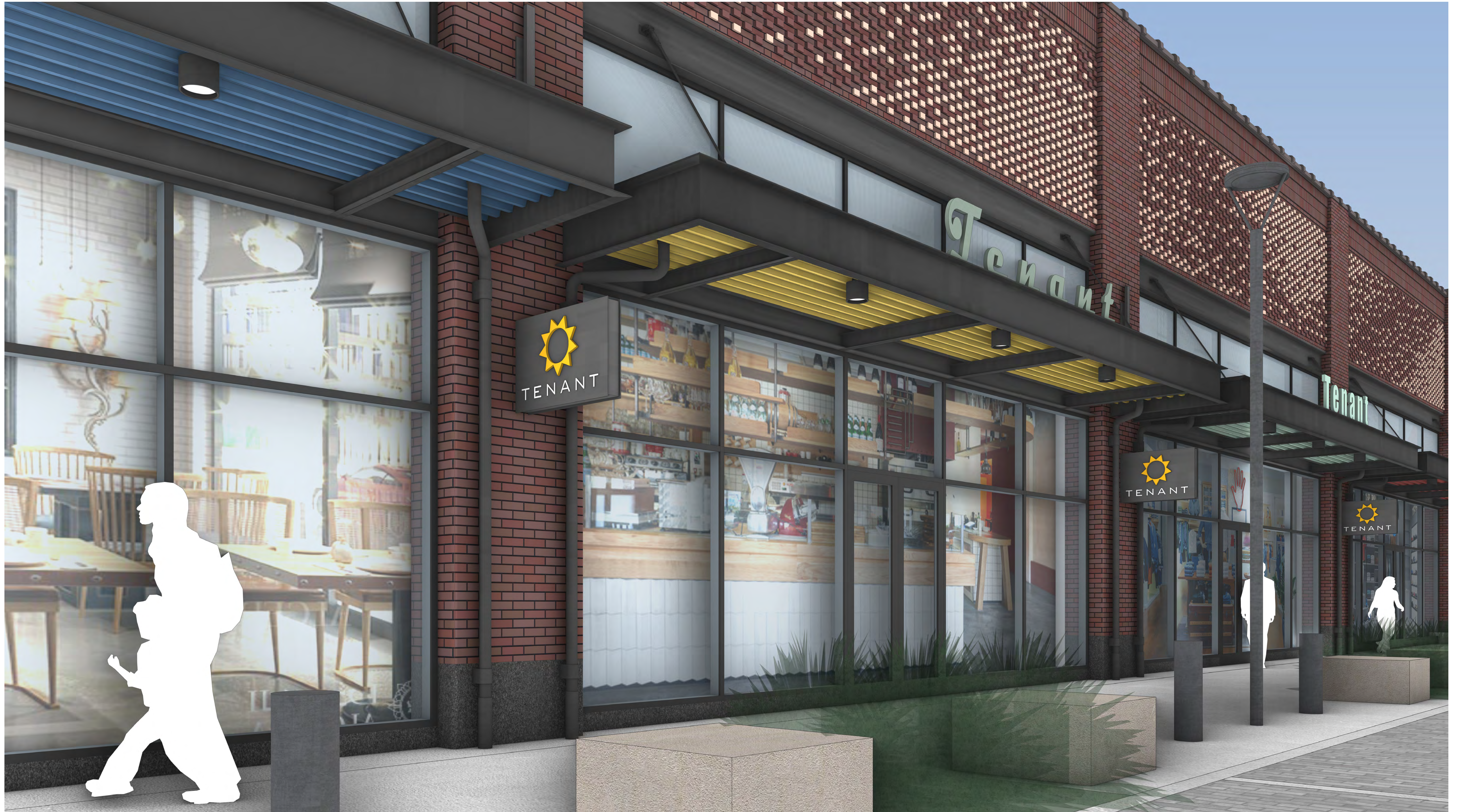
BUILDING 100 View of South Facing Canopy
