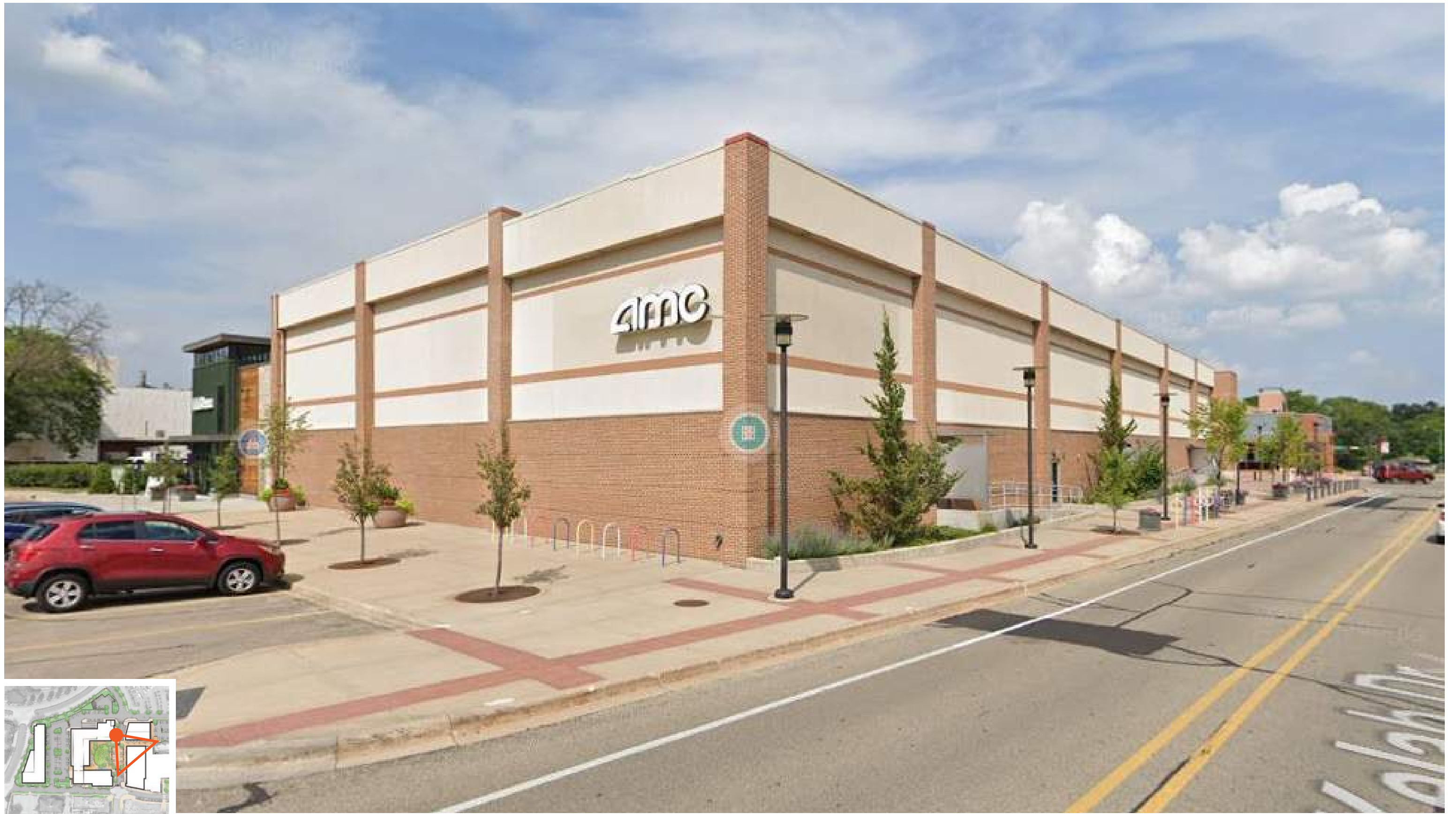
BUILDING 100 - SOUTHWEST PHOTO OF EXISTING
