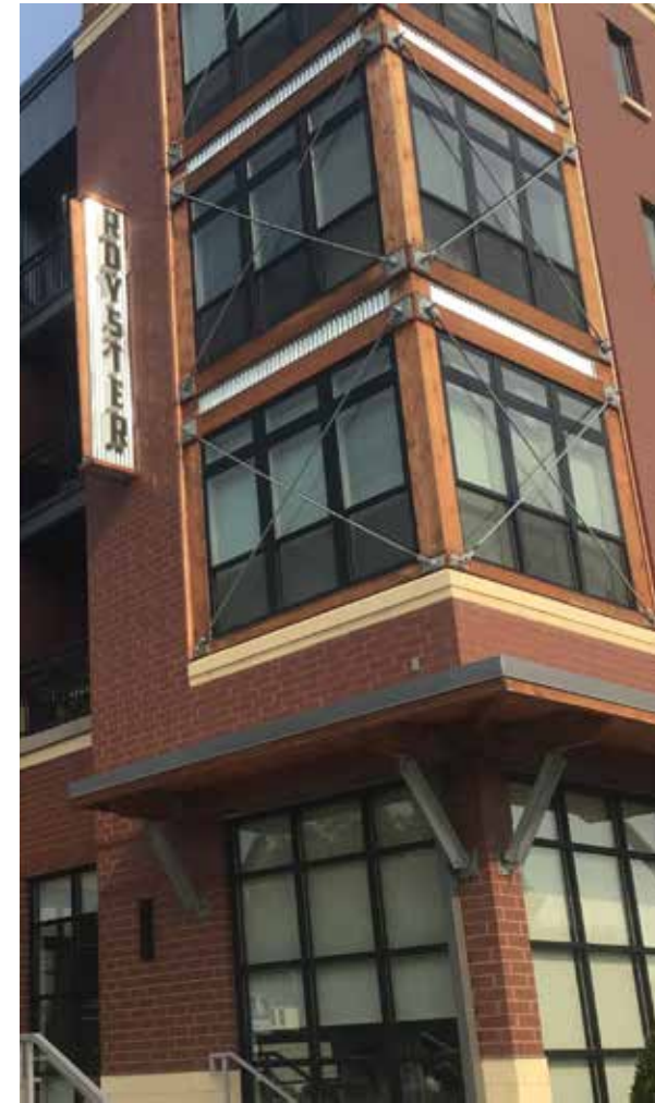
Projecting Sign Facing Cottage Grove Rd. Installed between 2 & 3 Floor
