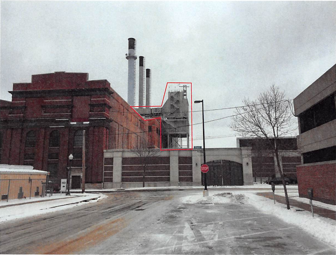
View from Railroad Street looking northeast.
