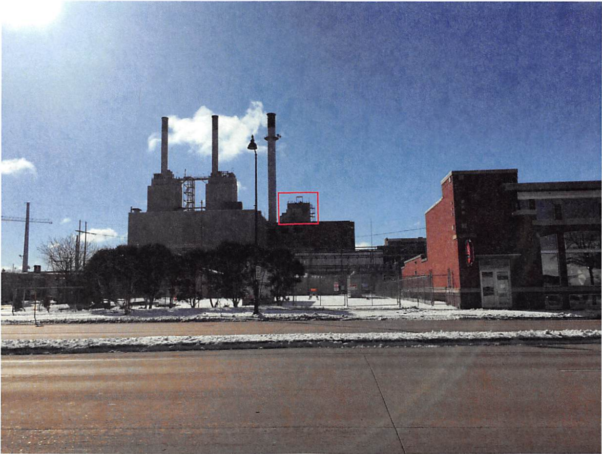
View from East Washington looking southeast.
