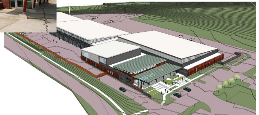
Nakoosa Fleet Facility
