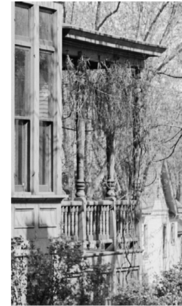
ORIGINAL PORCH RAILING
