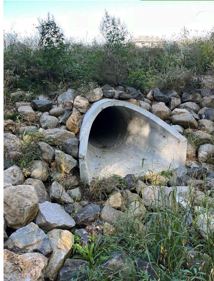
Outfall in dry weather
