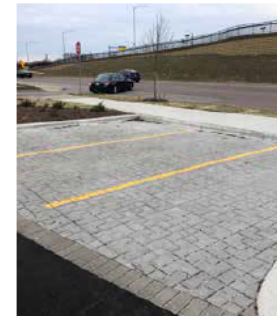
Pervious pavement at Portillos at West Towne.
