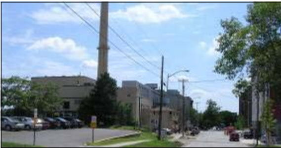
■ UW-Madison's Charter Street Heating and Cooling Plant.
