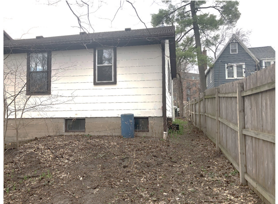
REAR VIEW, WEST SIDE. NEW DOOR OPENING, LANDING AND STAIR TO GRADE HERE
