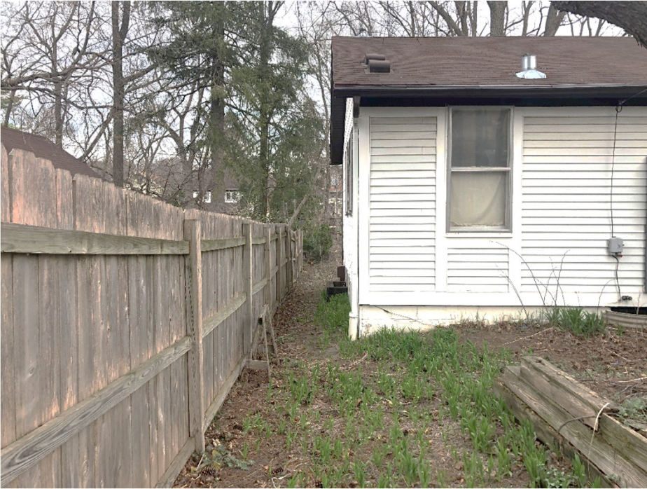
FRONT VIEW, WEST SIDE
