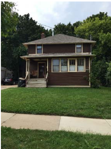
306 Lathrop, Front – East Elevation
