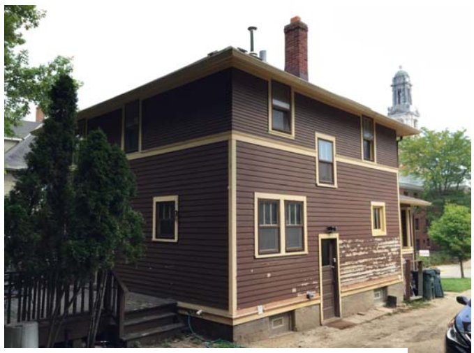
306 Lathrop, Side – Southwest Elevation
