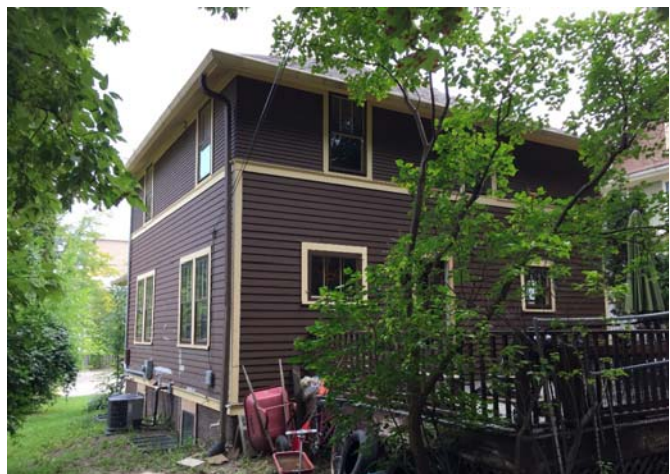
306 Lathrop, Northwest Elevation
