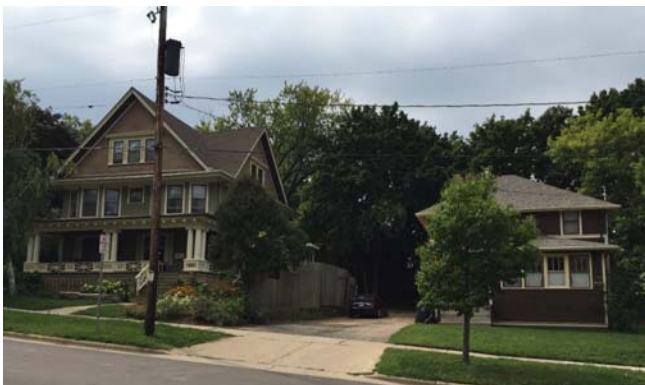
302 Lathrop on Left, 306 Lathrop
