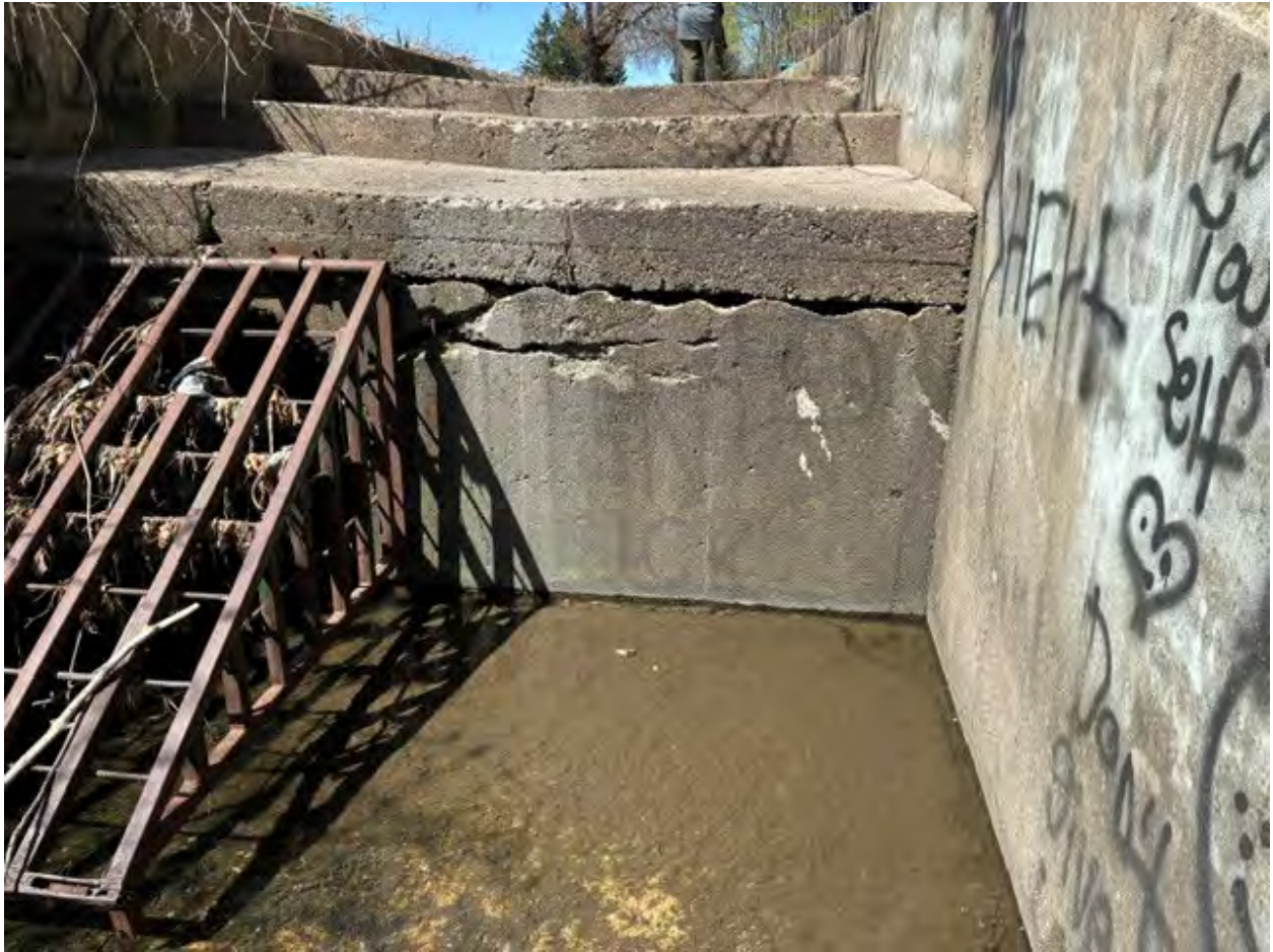
Central Drop Structure – Provide New Gate, Under-Pipe Repair & Void Repairs
