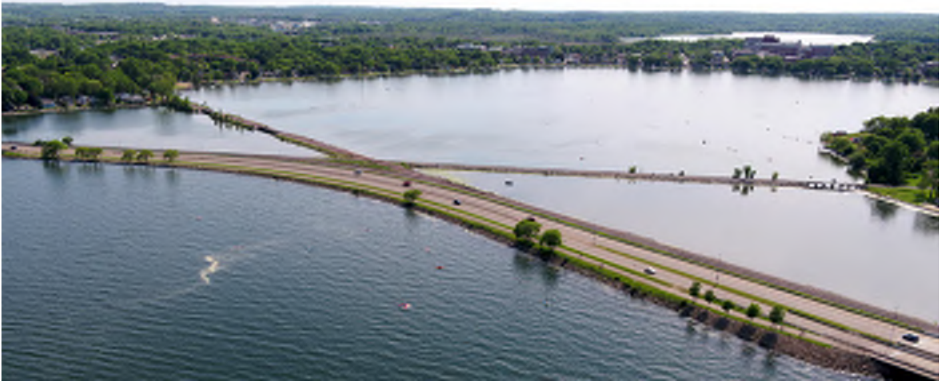
Figure 4 John Nolen Drive Causeway View Looking Southwest
