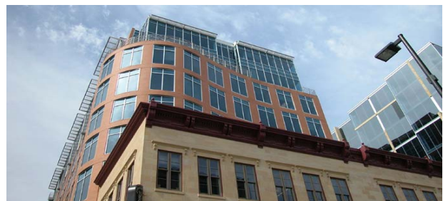
Block 89 Office Development
