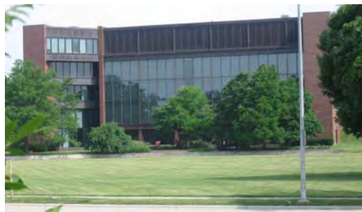
Office use across Mineral Point Rd.
