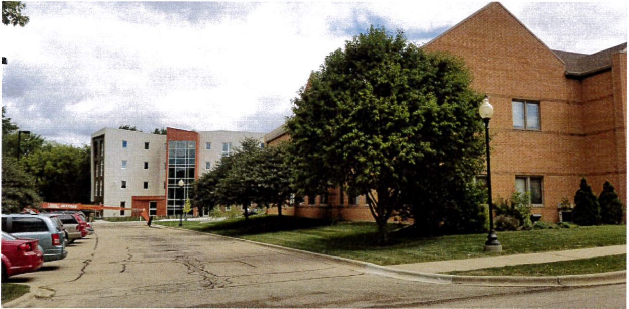
VIEWING NORTH FROM SOUTH ACCESS ROAD
