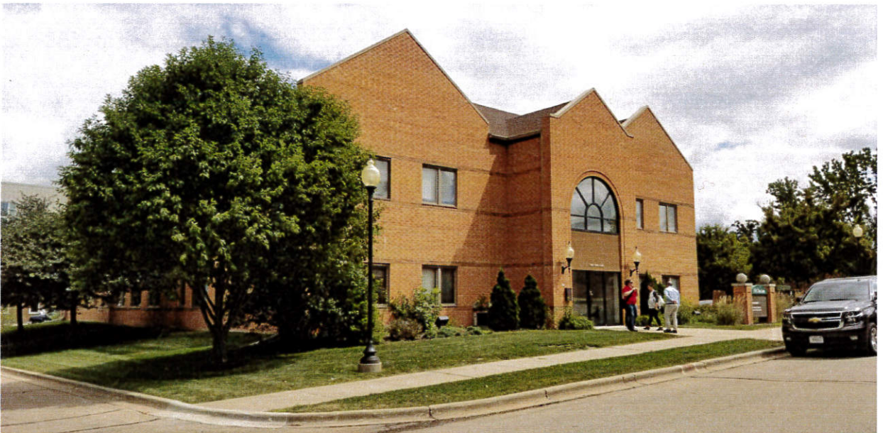
VIEWING NORTHEAST FROM SOUTH ACCESS ROAD
