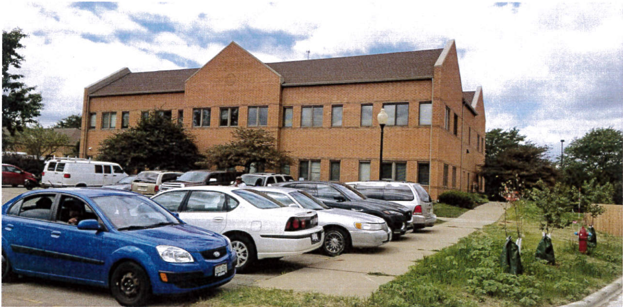
VIEWING NORTHWEST FROM EAST ACCESS DRIVE
