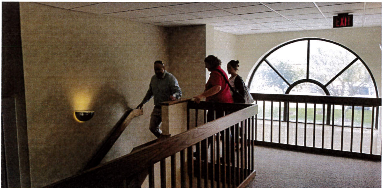
VIEWING SOUTH - SECOND FLOOR LOBBY
