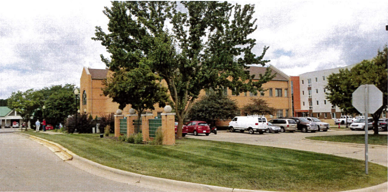
VIEWING NORTHWEST FROM SOUTH ACCESS ROAD
