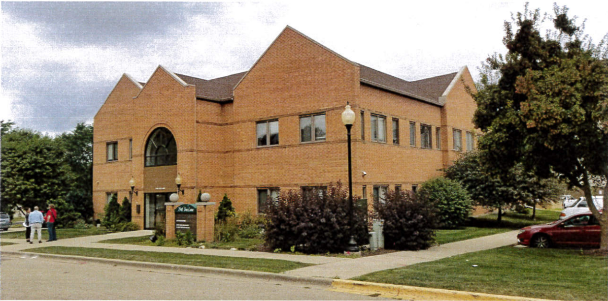
VIEWING NORTHWEST FROM SOUTH ACCESS ROAD
