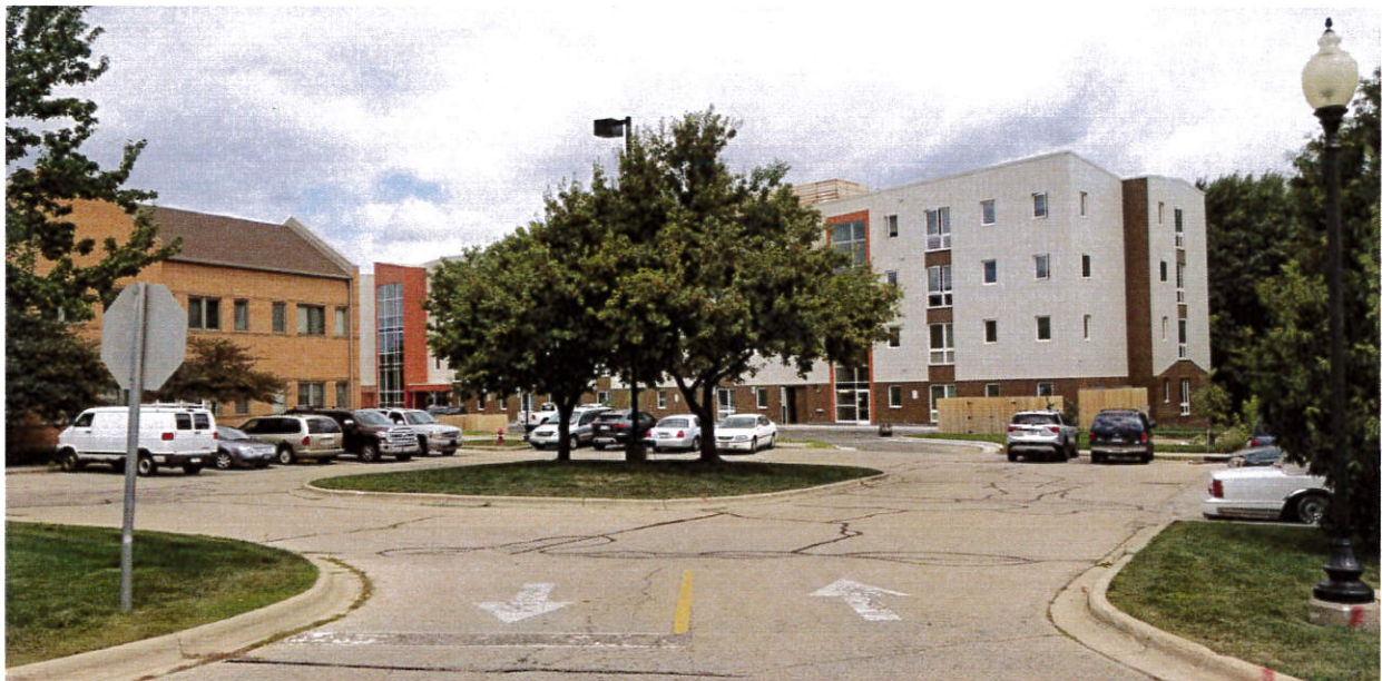
VIEWING NORTH FROM EAST ACCESS DRIVE
