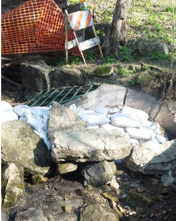
Erosion at the upstream storm sewer caused by failure of the diversion wall
