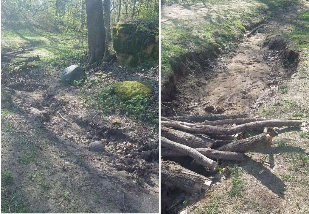
Erosion Downstream of Existing Inlet
