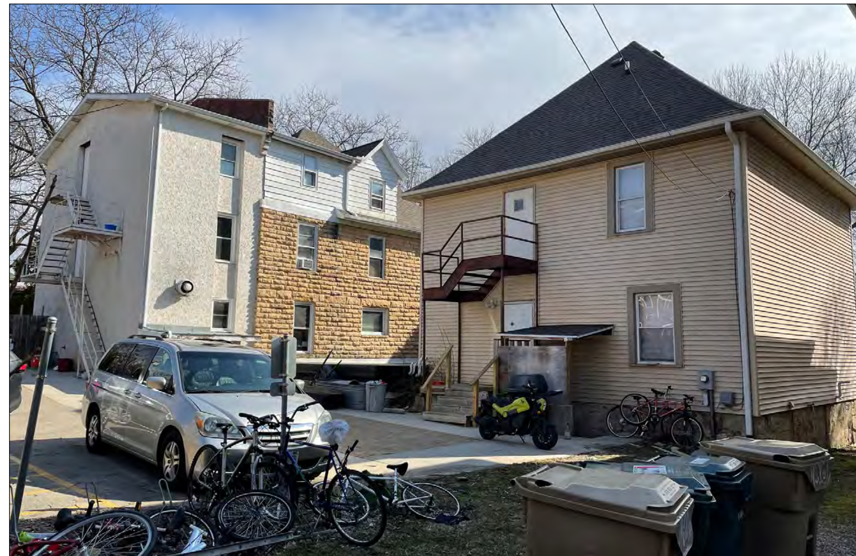
REAR OF THE BUILDINGS AT SOUTH WEST CORNER OF THE PROPERTY
