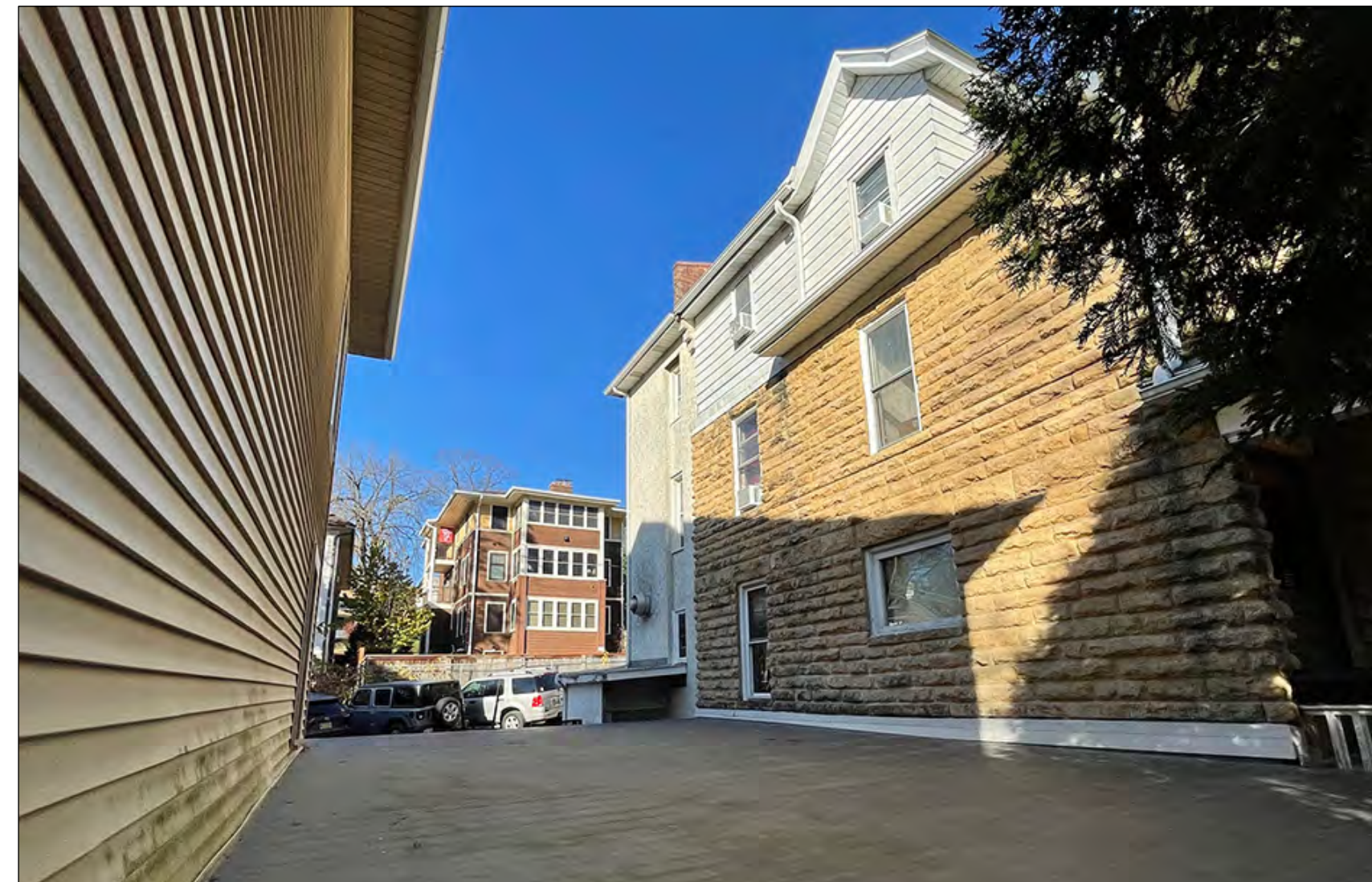
1ST FLOOR: ROOF OF LOWER LEVEL BUILDING CONNECTION
