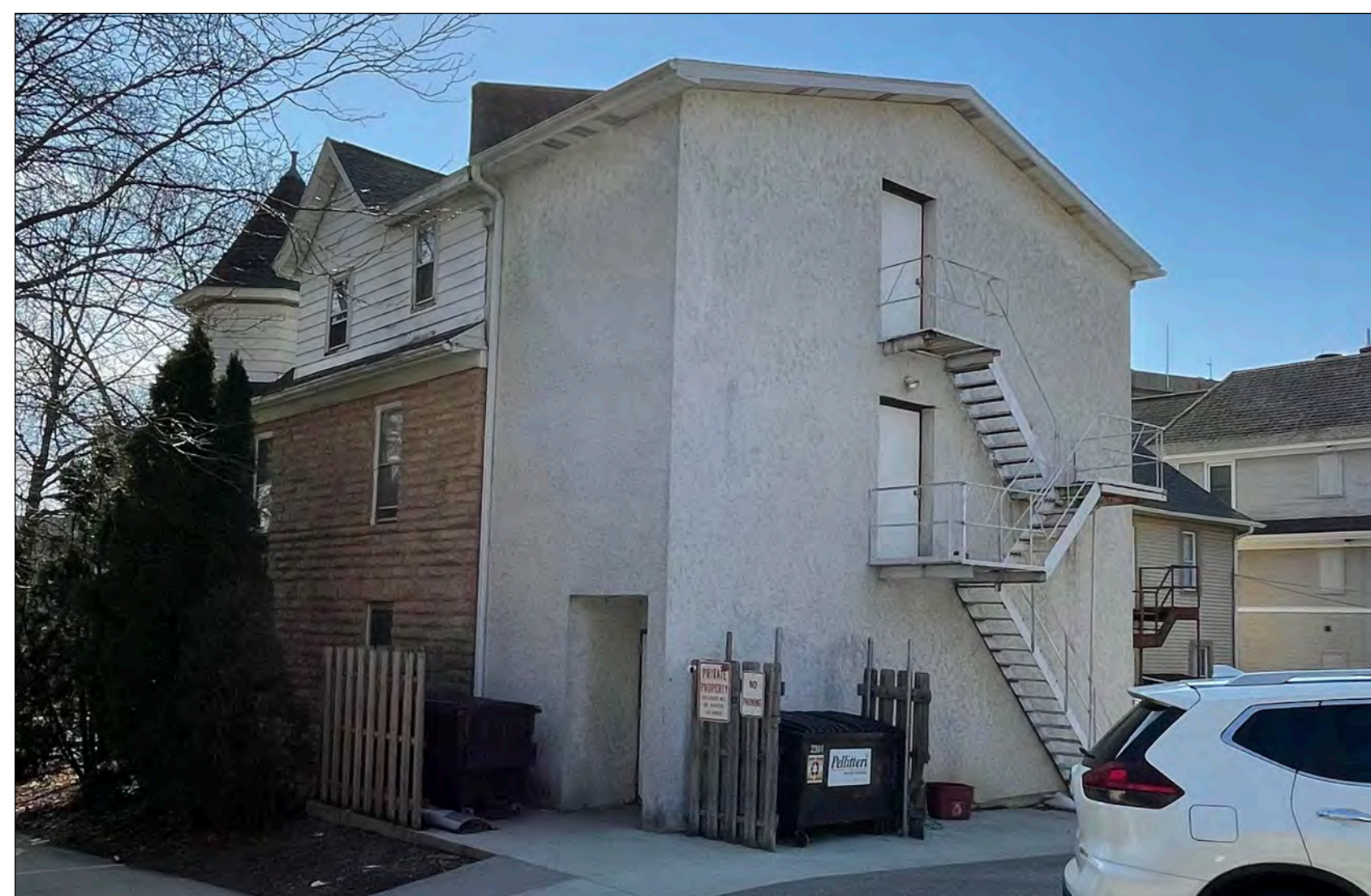
REAR ELEVATION OF THE 148 BUILDING
