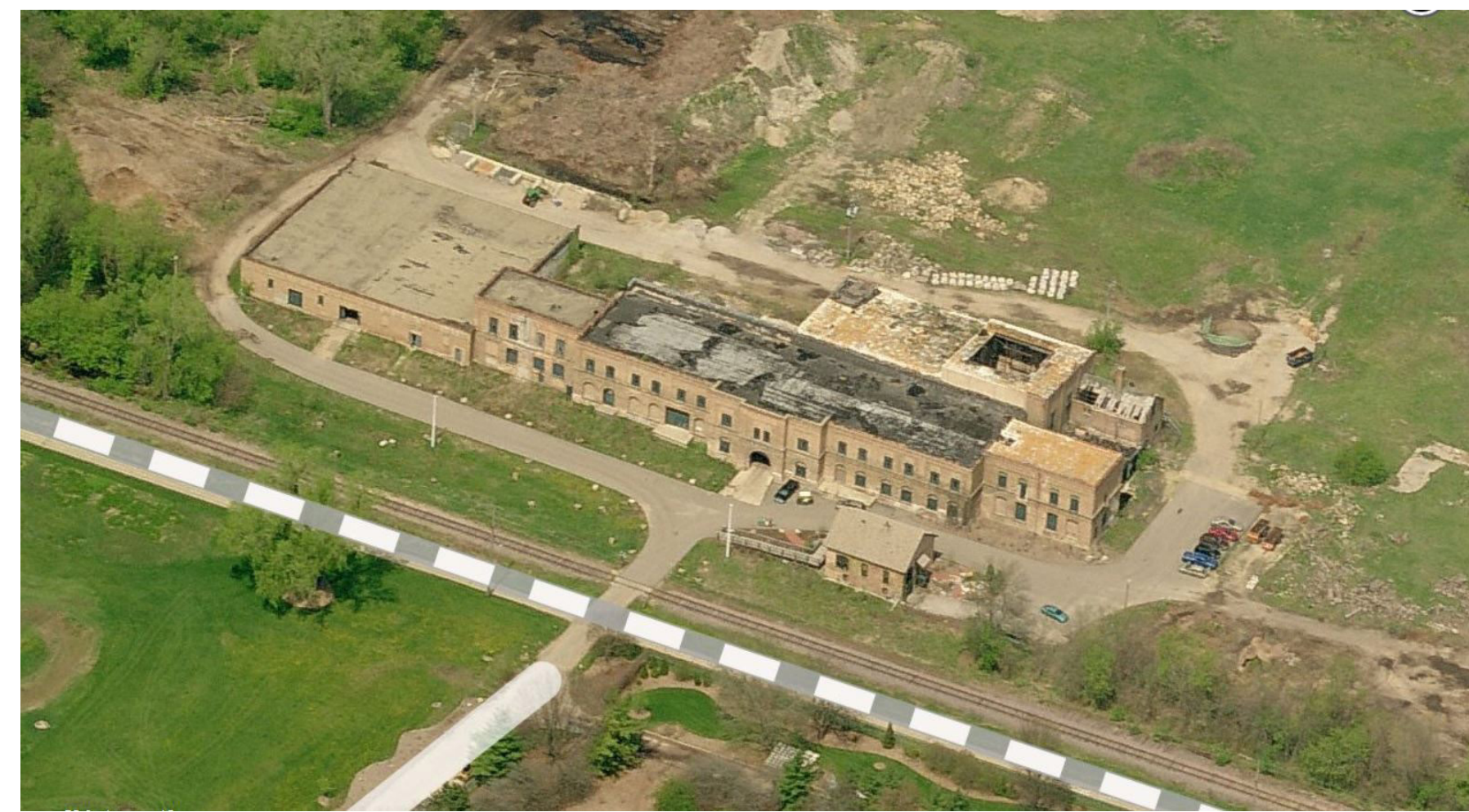
EXISTING SOUTH FACADE AERIAL
