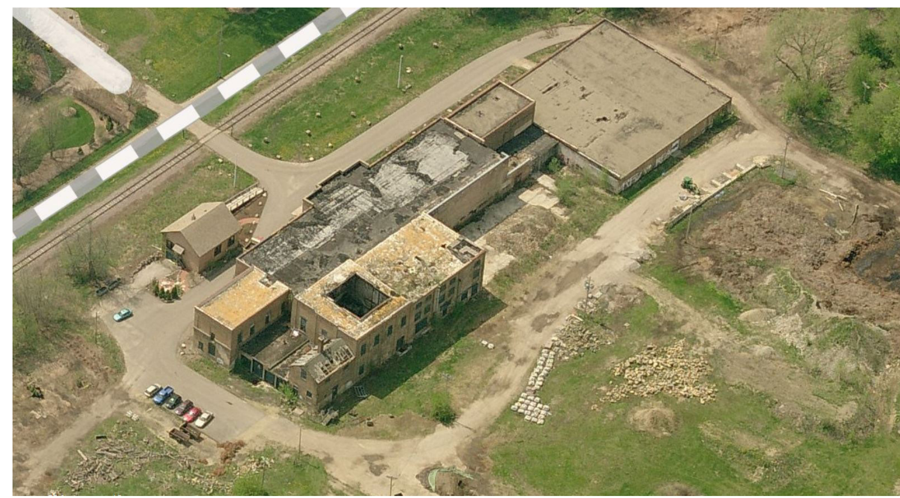
EXISTING NORTH FACADE AERIAL
