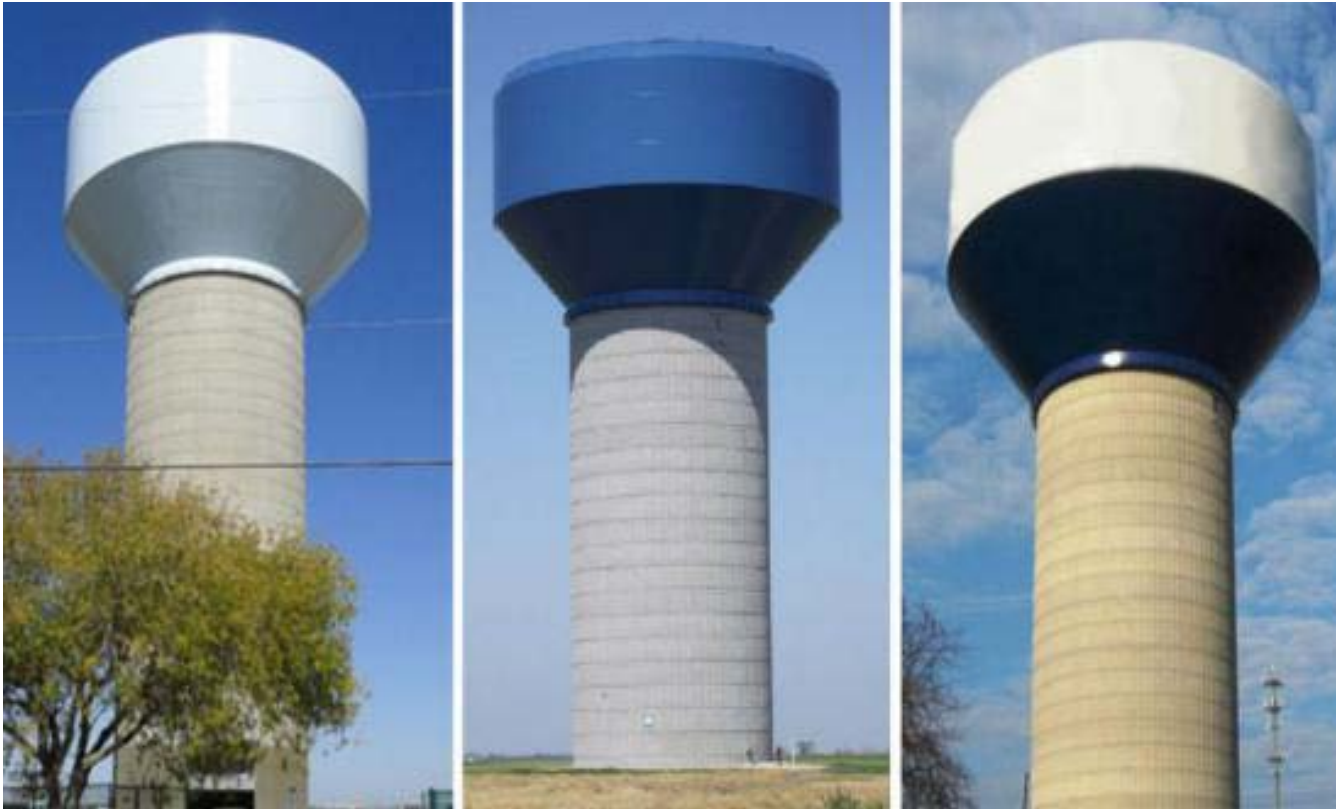
Single or Two Toned Tank Paint Examples for Composite Tank
