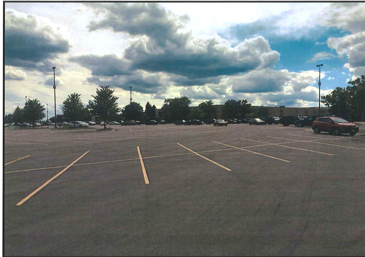
Existing Parking Lot and Building from the North
