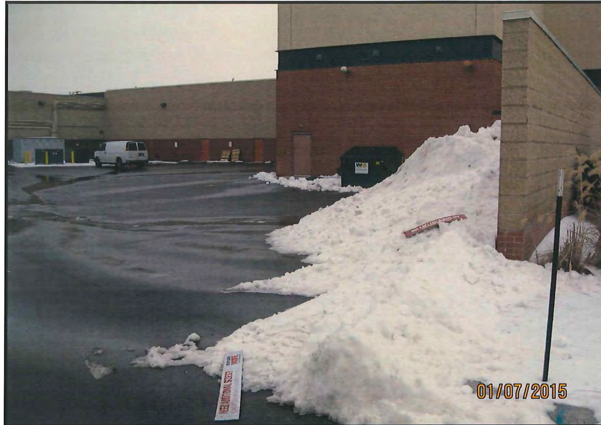
Maintenance Access and Snow Storage
