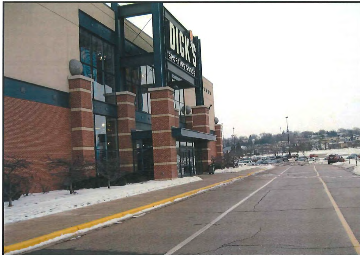
Facade of Adjacent Building to the North
