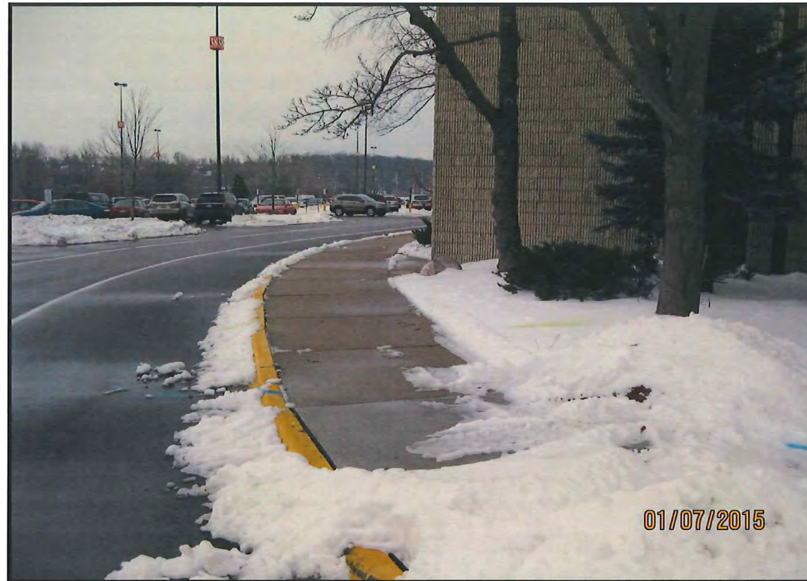
Fire Access Continued to Adjacent Building to the North
