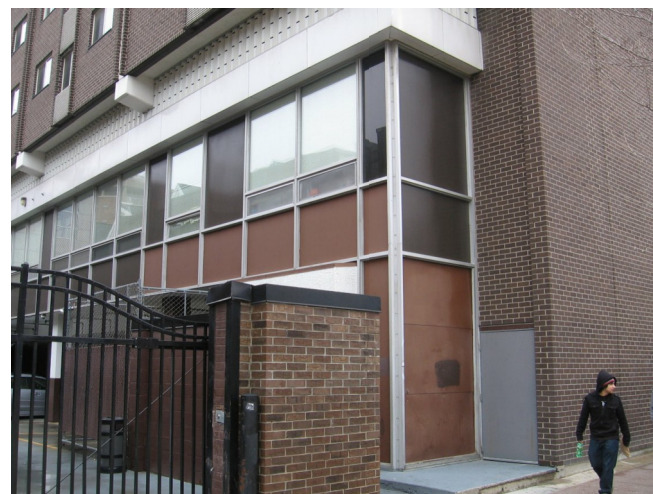
EXIT FROM EGRESS STAIR
