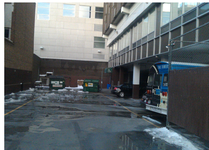
EXISTING PARKING LOT
