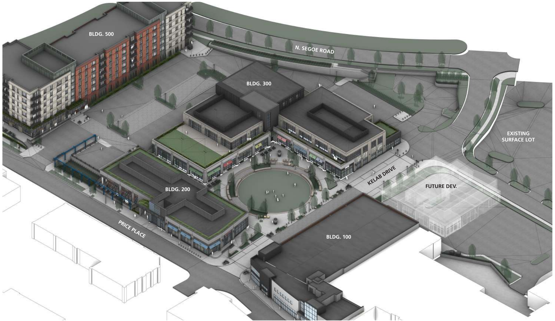
HILLDALE PHASE 3 View Looking Southwest
