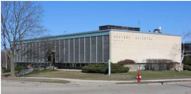
Grayson Building 4414 Regent Place
