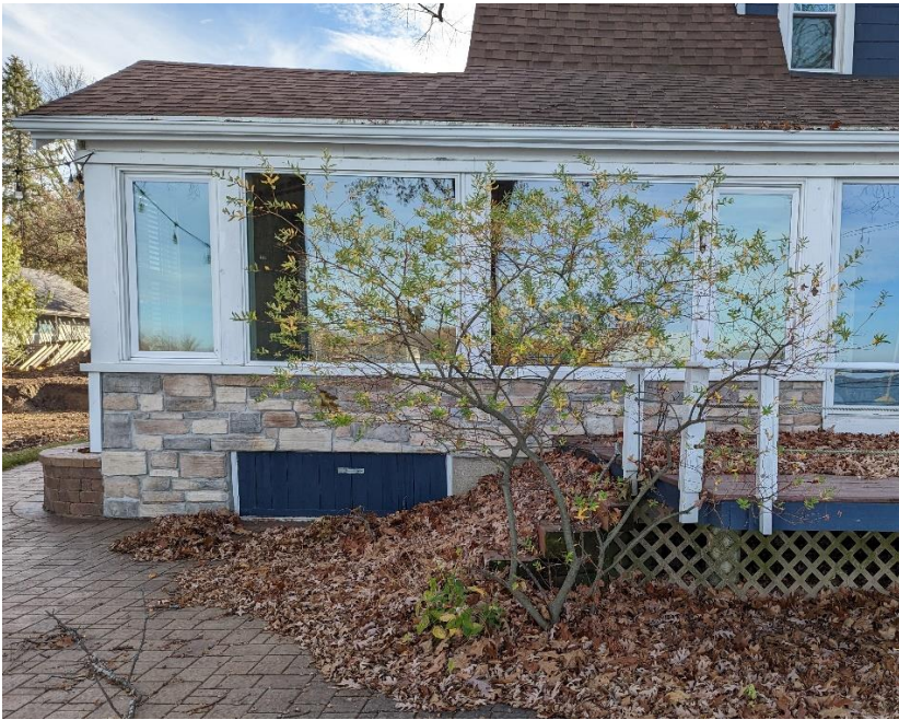
Lake Side of House – The upper windows are non historic vinyl inserts, deck is deteriorating and near end of life. Roof ridge shows sagging structure and settling of foundation.
