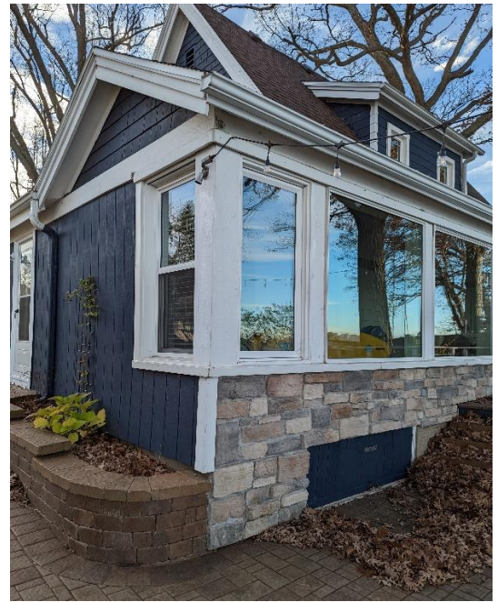
Lake Side of House – The upper windows are non historic vinyl inserts, deck is deteriorating and near end of life. Roof ridge shows sagging structure and settling of foundation.
