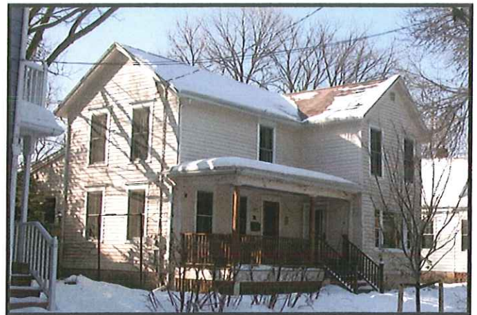
414 S. Few St. (built 1880) [1518 sq.ft.] Precedent for Farmhouse Vernacular Style
