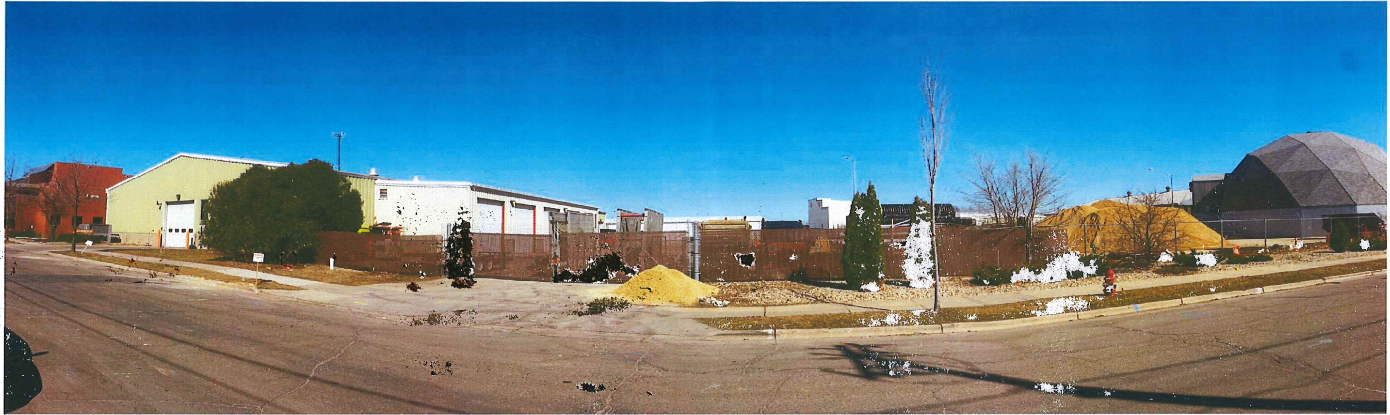
Existing View from South
