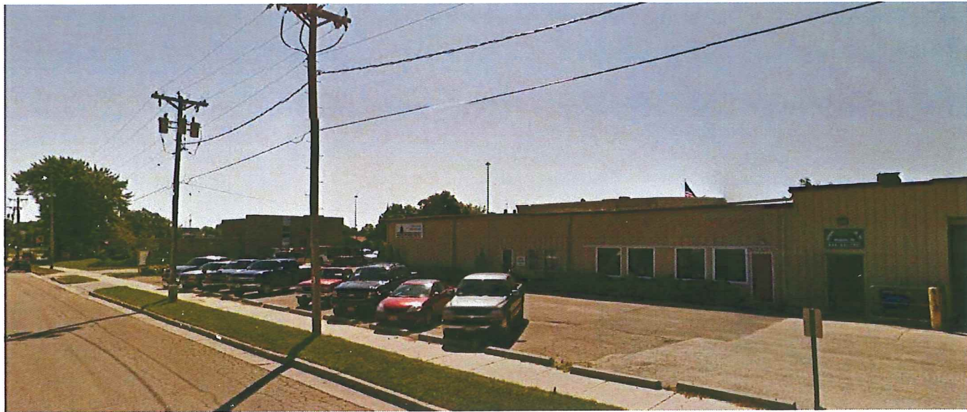
View to SE across Emil St.
