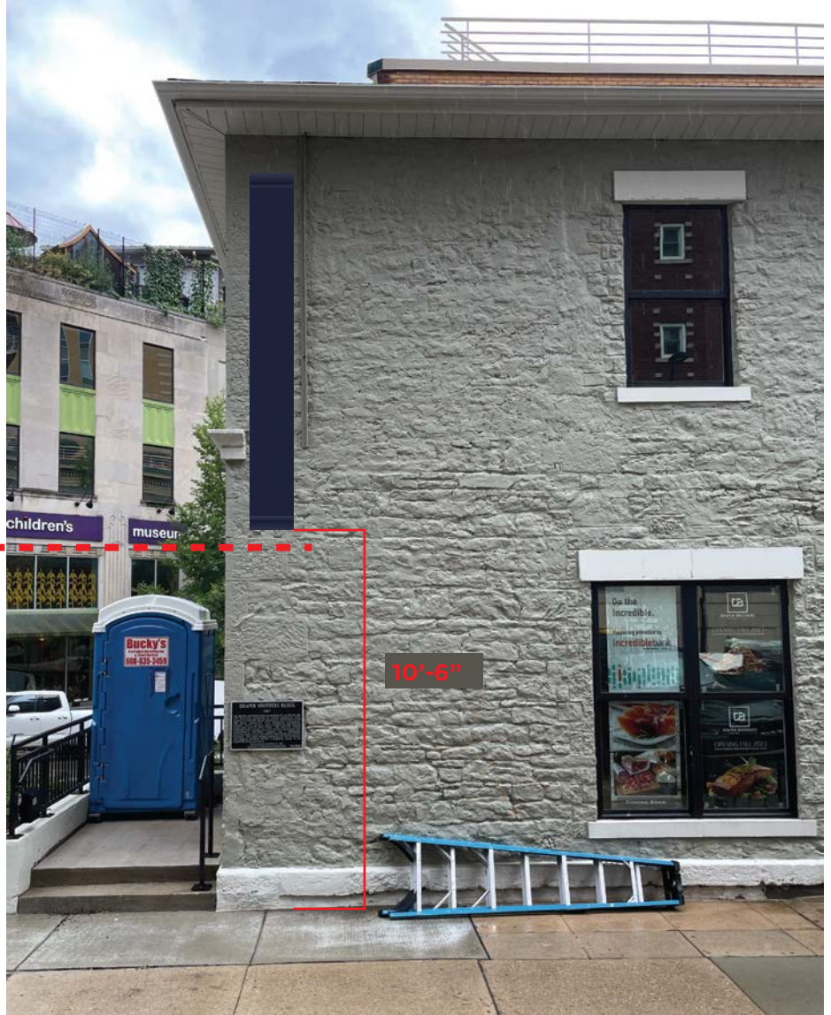
FACING NORTH ON E. MIFFLIN ST. TOWARDS 101 N. HAMILTON
