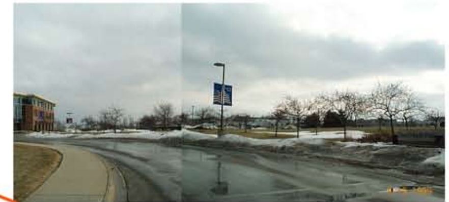
View S along the E entry drive to the main building with the new parking area at center right
