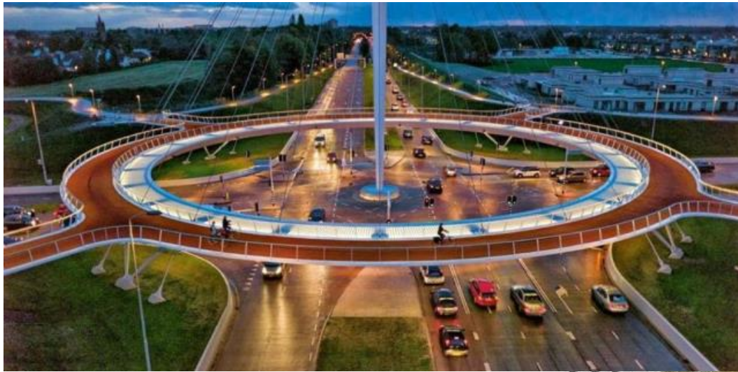
Hovenring, Eindhoven, Netherlands (designed by ipv Delft)
