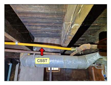
**5.5** (2) **Defect:** A gas supply line was shut off at the valve but was not capped. If the valve is opened, gas will flow into the home and create a dangerous condition.
