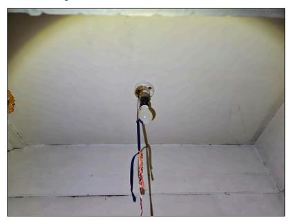
**6.4** (3) **Defect:** In multiple rooms, there was not a way to turn on a light when entering a room through a doorway.
