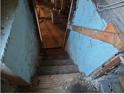
(2) **Defect:** A door opens over stairs without a landing being present. This is a fall hazard.
