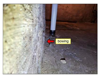
**4.2 Defect:** Columns were not constructed in a manner or in a condition to adequately support the floor structure.
