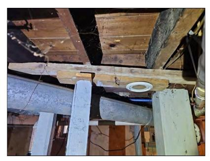
**4.3 Defect:** Joist(s) were altered in a manner that impact their structural integrity. Main beam was resting on chimney corbels - cracks were present. Please see note 1.4 about the condition of the bottom of the chimney. Subfloor was deteriorated.
