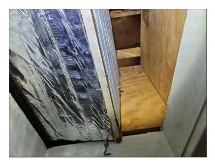
**4.5 Further Evaluation:** The attic hatch was covered in foam board insulation. After repeated attempts, the Inspector was not able to raise the hatch completely - it was bumping into the roof decking.
