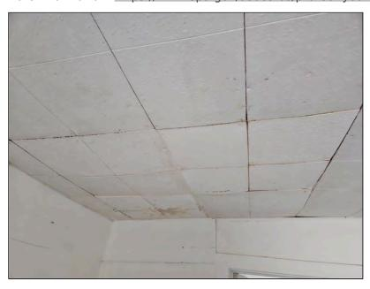
**3.0** (2) **Repair:** The plaster was disengaged/cracked in multiple locations. Recommend further evaluation and repair as necessary by a qualified contractor.
