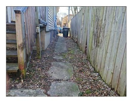
**2.6 Repair:** The landscaping was insufficiently sloped away from the home in multiple locations. This can cause excessively high levels of moisture at the foundation and cause damage to the foundation and moisture intrusion into the basement. Recommend correcting landscape to drain water away from home.
