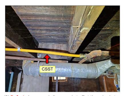
(2) **Defect:** A gas supply line was shut off at the valve but was not capped. If the valve is opened, gas will flow into the home and create a dangerous condition.
