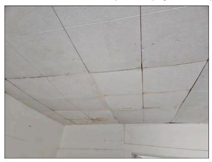
(2) **Repair:** The plaster was disengaged/cracked in multiple locations. Recommend further evaluation and repair as necessary by a qualified contractor.
