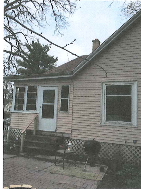
View From the North Side
