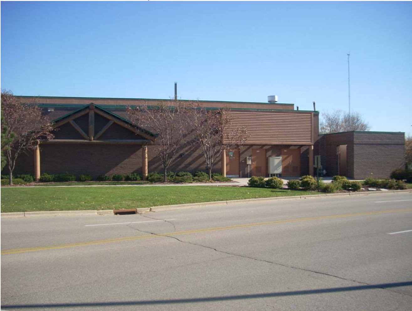
4) View – east, from JCP parking lot (panoramic)
