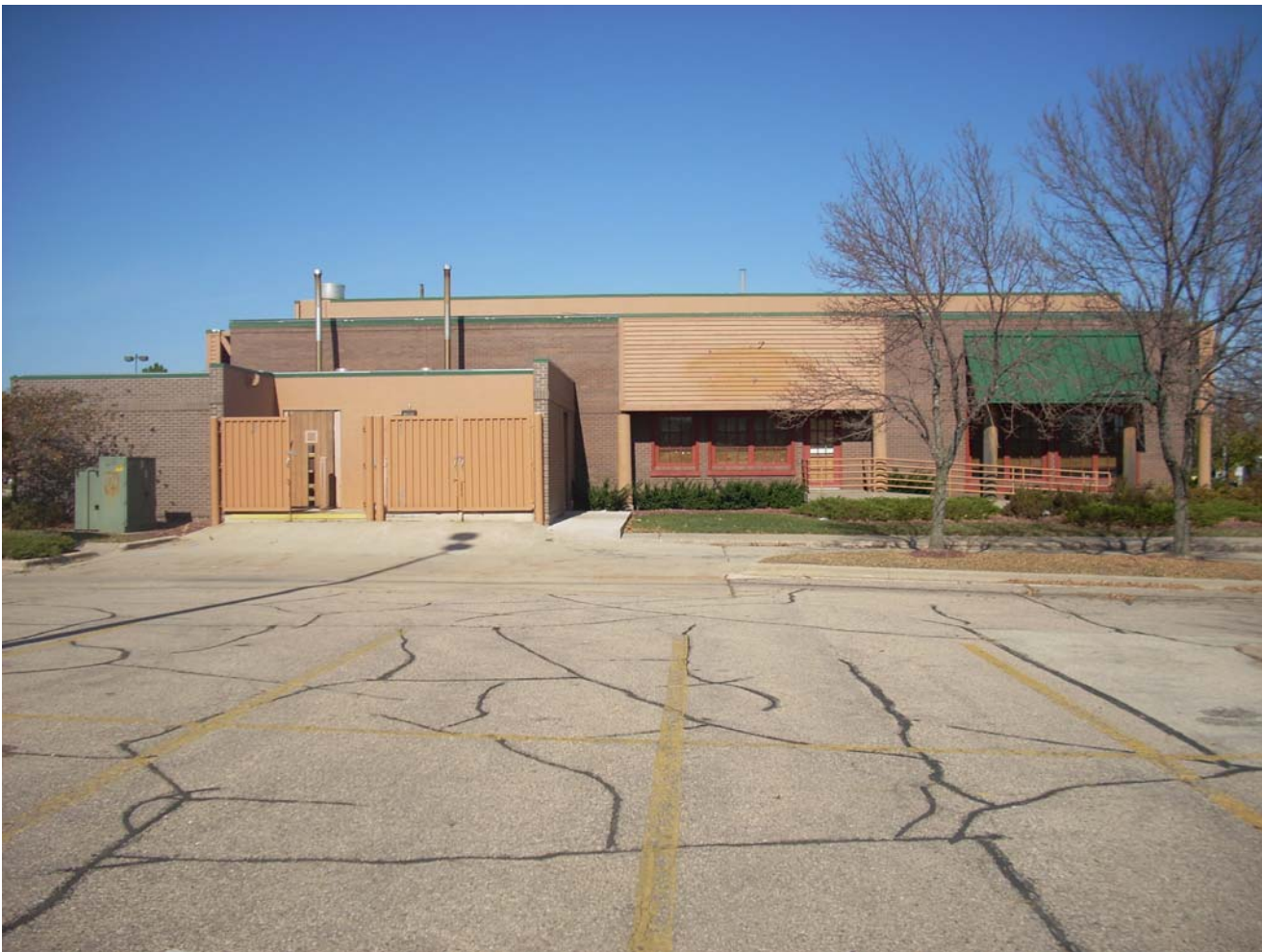
2) View – north, wall faces Mall entrance drive
