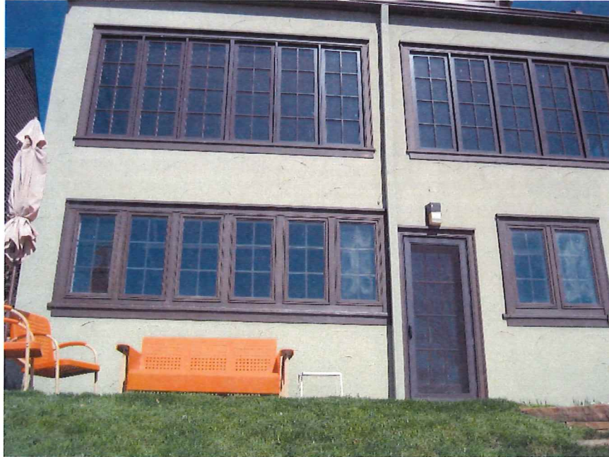
1. Current windows and “short” door to allow clearance with boiler pipers inside
