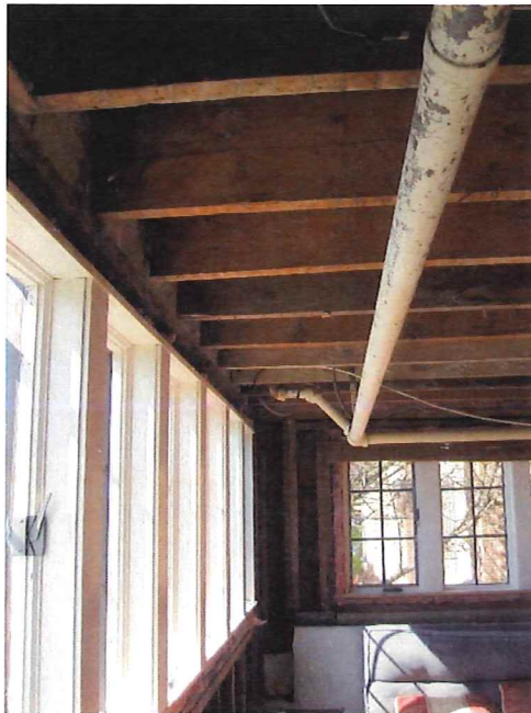
2. And 3. Boiler pipe is ~19” from lakeside wall thus restricting inward swinging hinged door.
